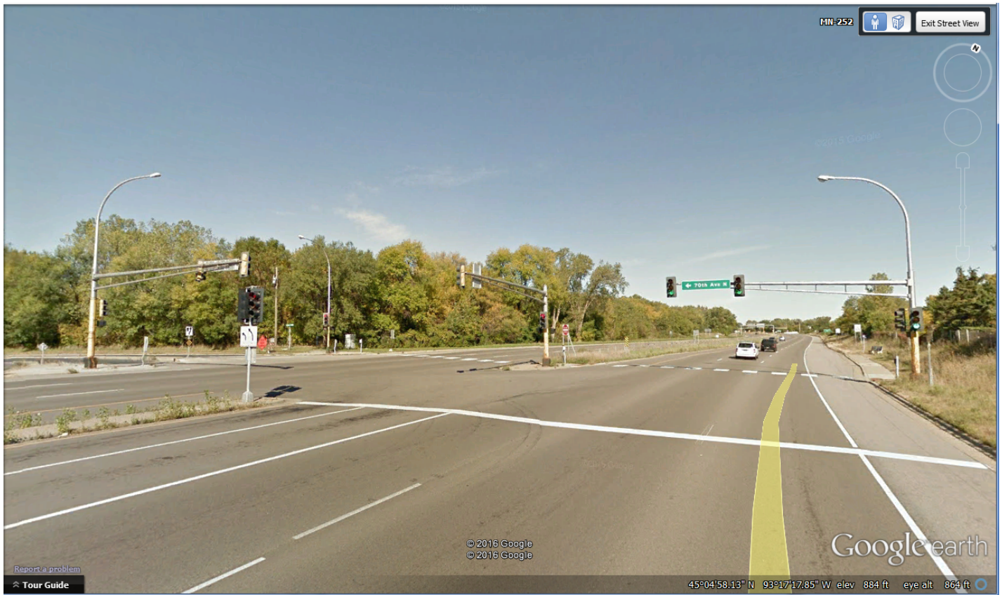
TH 252 at 70 th Avenue N – looking north
