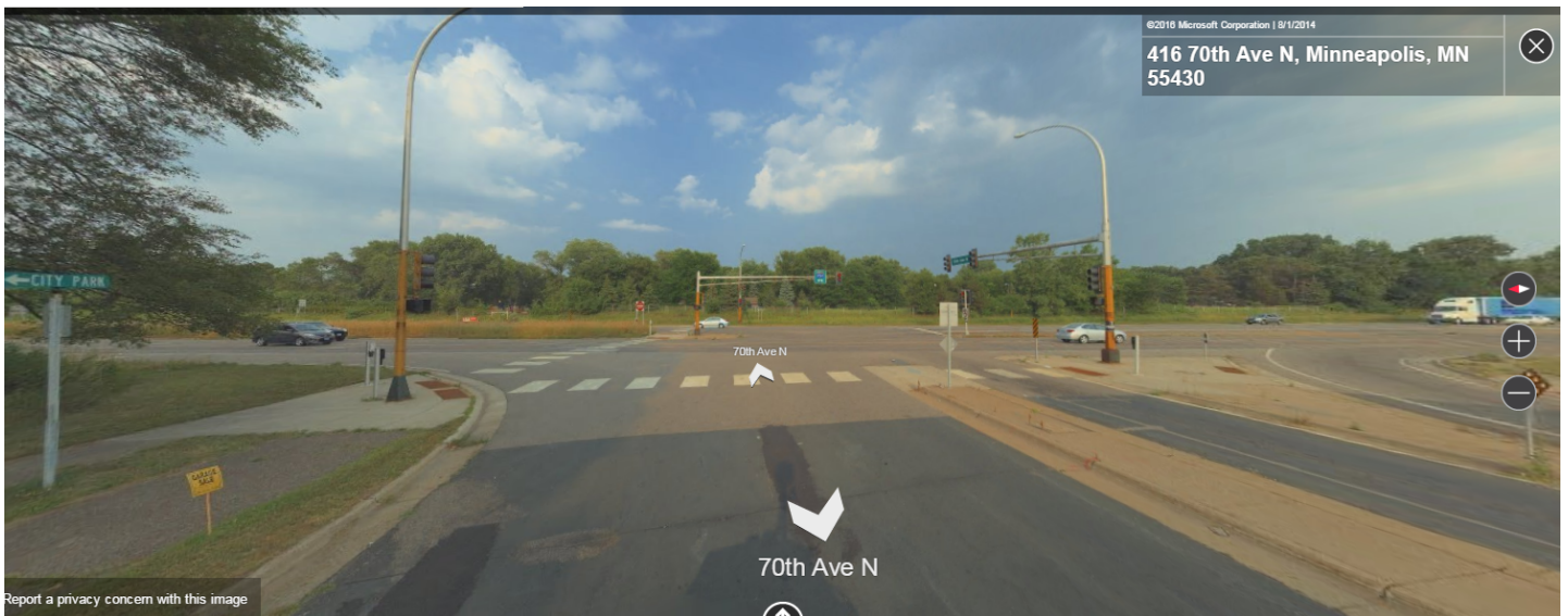
TH 252 at 70 th Avenue N – looking west
