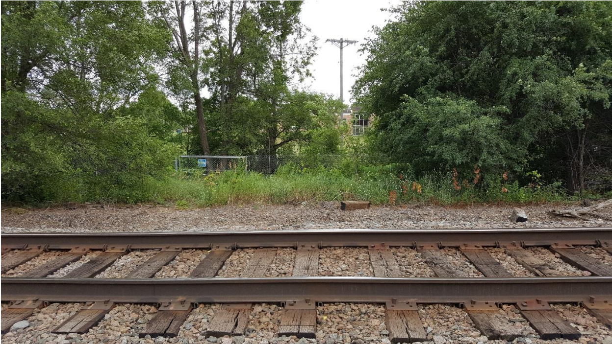
BNSF Railway near Edgewood Avenue – looking South towards Hobart Elementary
