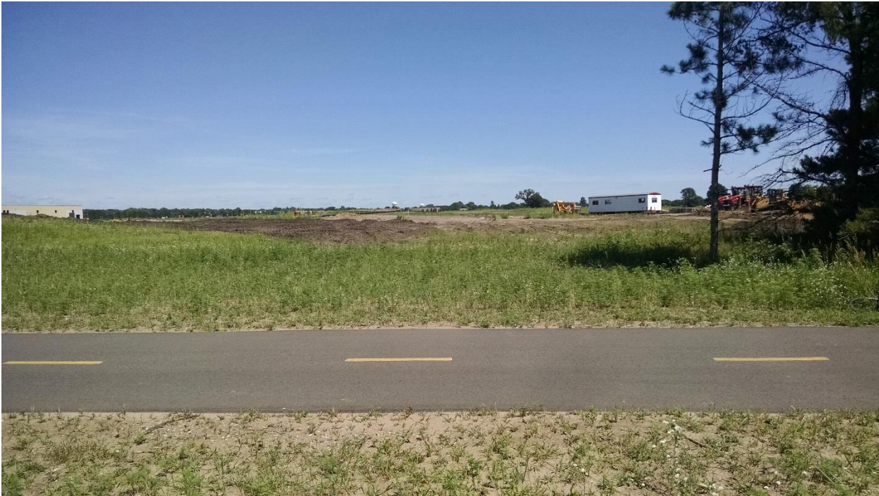
Rush Creek Trail – Future Xylon Avenue Crossing – View from south of crossing looking north. NorthPark Business Park currently under construction.
