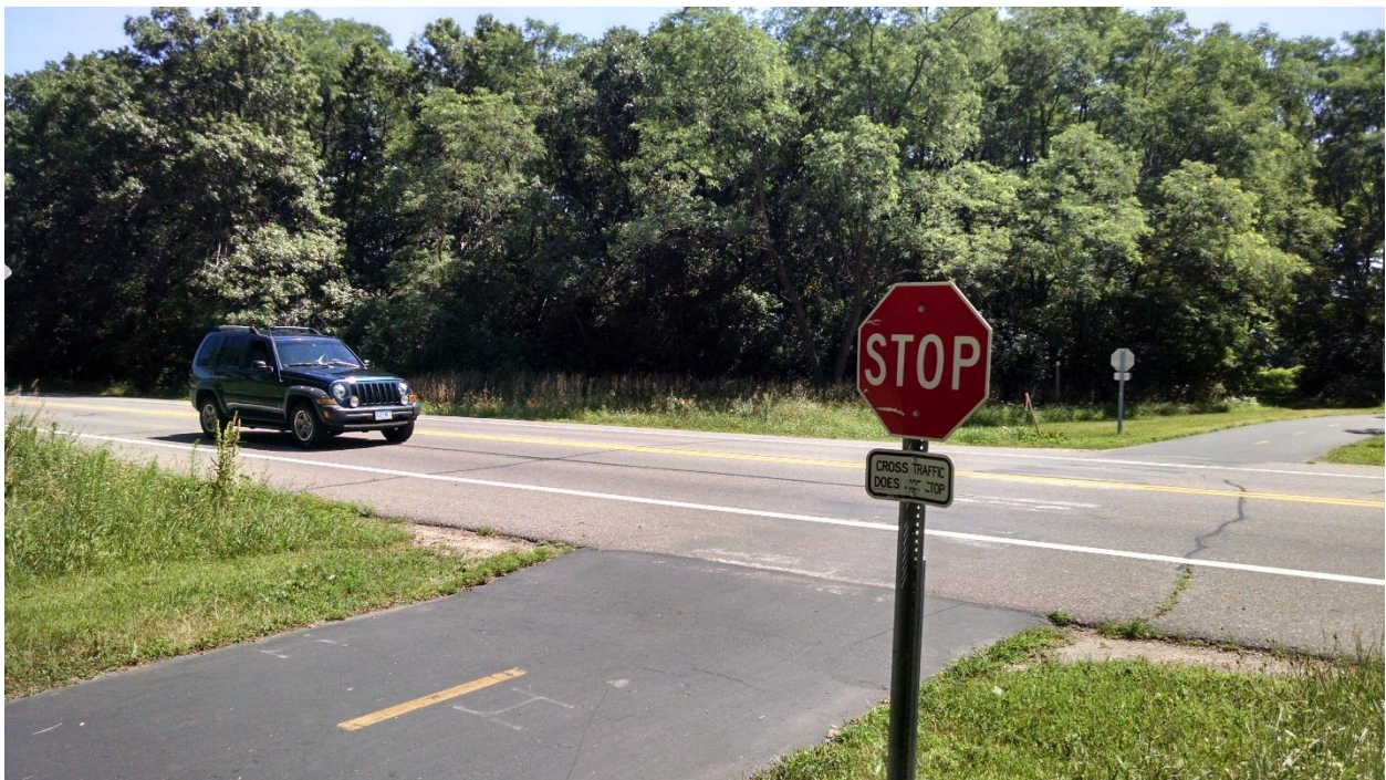
Rush Creek Trail – Winnetka Avenue North Crossing – View from southwest of crossing looking northeast.
