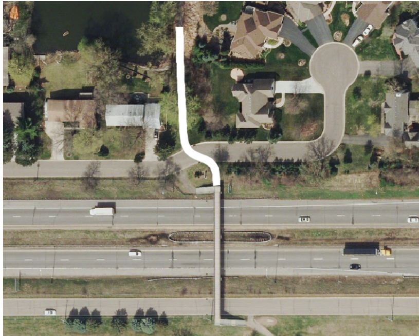
Figure 13: Example of “Flyover” Bridge Connecting into Existing Bike Path
