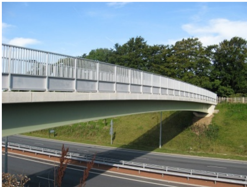
Figure 5: Example of a Slab/Girder Pedestrian Bridge
