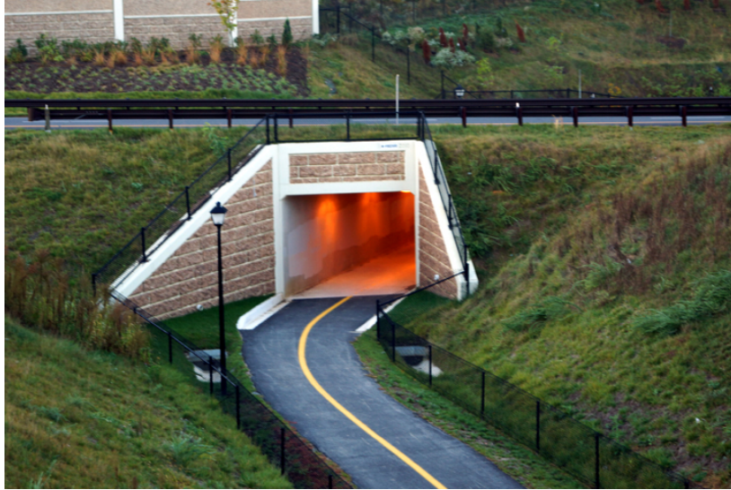
Figure 16: Example of Bike Tunnel underneath Highway
