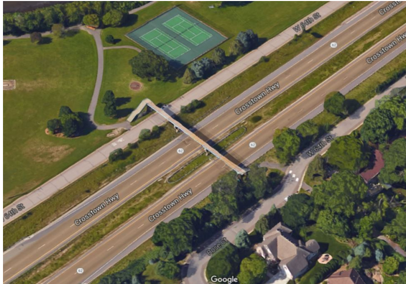
Figure 2: Aerial View of Current Bridge and Surrounding Area
