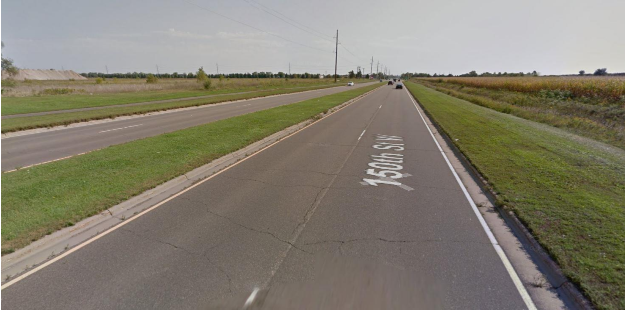
CSAH 42 facing east at proposed underpass location
