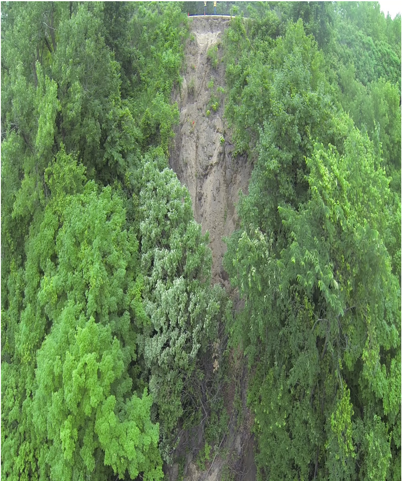
Trail damage immediately after storm event
