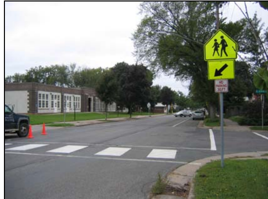
High-visibility crosswalk marking at Hiawatha School
