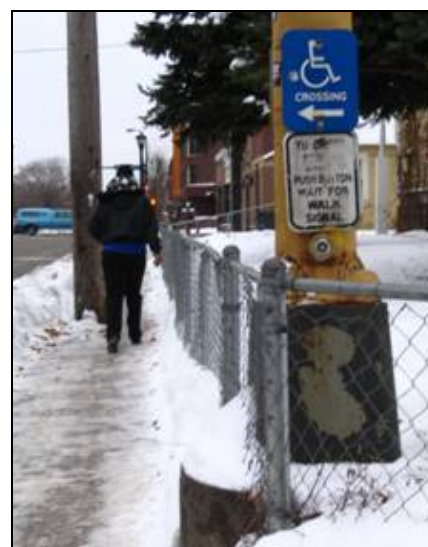
This push button is not accessible or convenient for all pedestrians.
