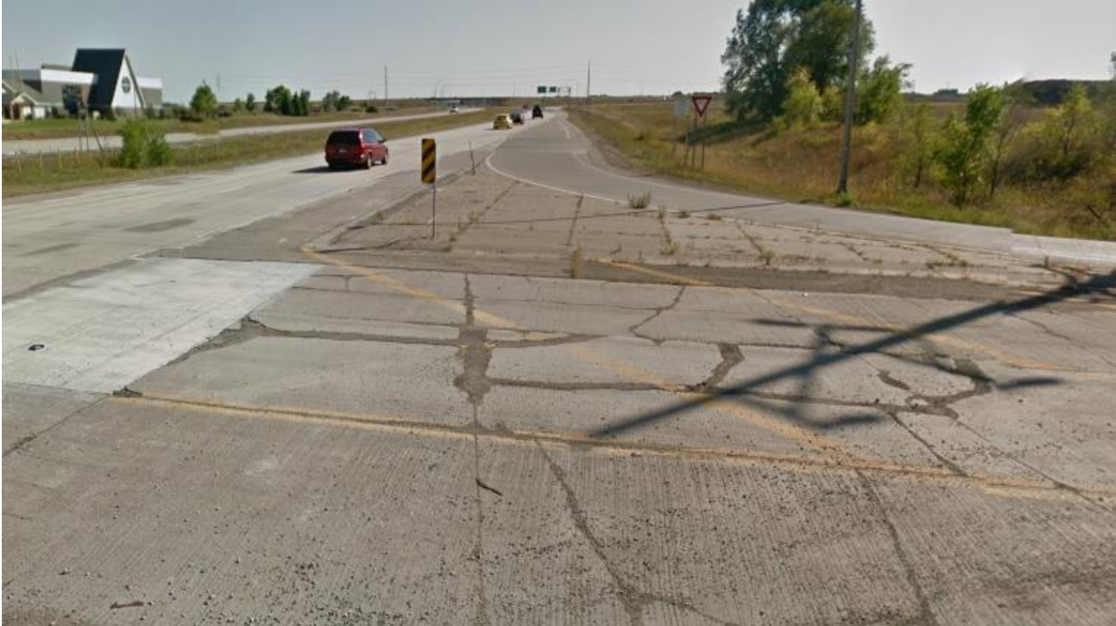
101 st Avenue North – From northwest looking south at US Hwy 169.
