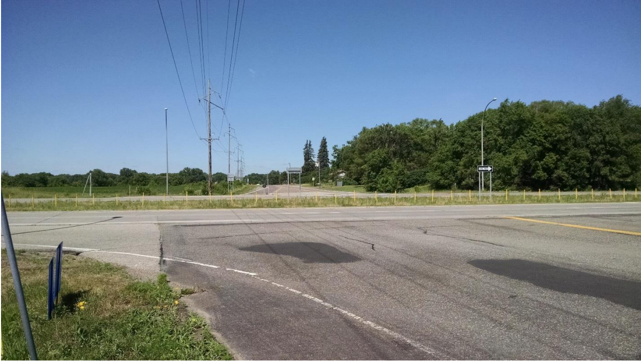
101 st Avenue North – From southeast looking west at US Hwy 169.
