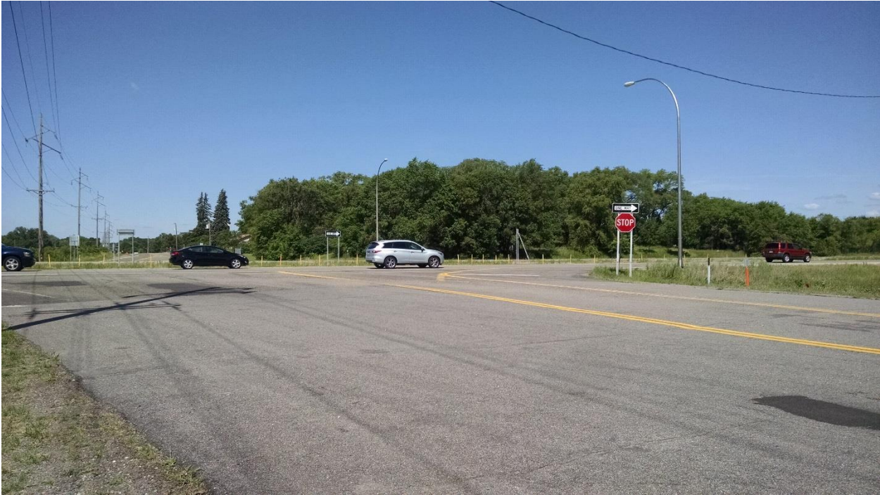
101 st Avenue North – From southeast looking northwest at US Hwy 169.
