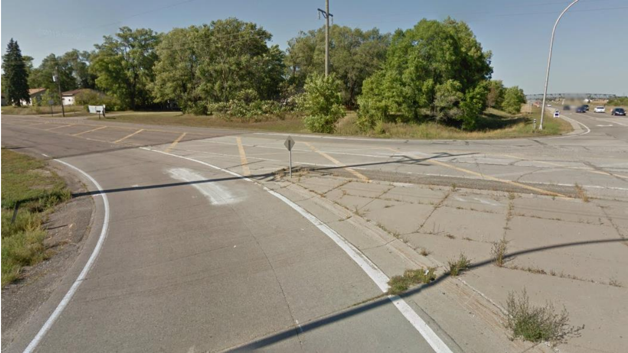
101 st Avenue North – From southwest looking north at US Hwy 169.
