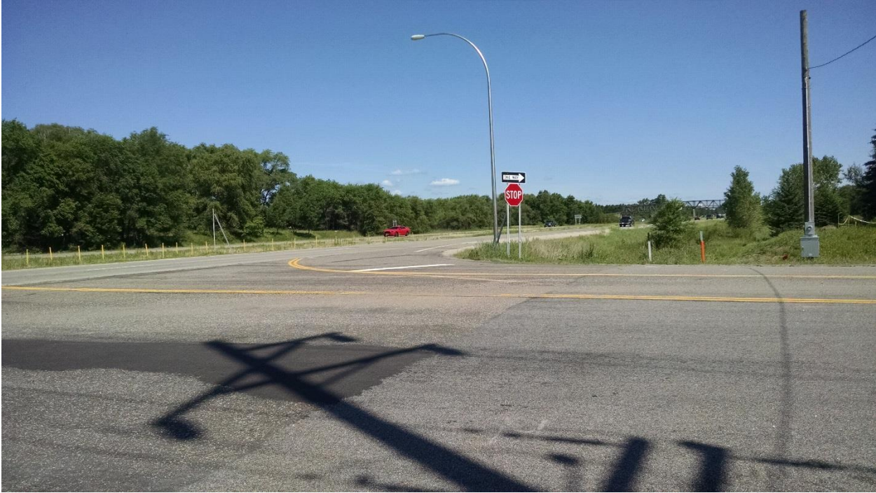
101 st Avenue North – From east looking northwest at US Hwy 169.
