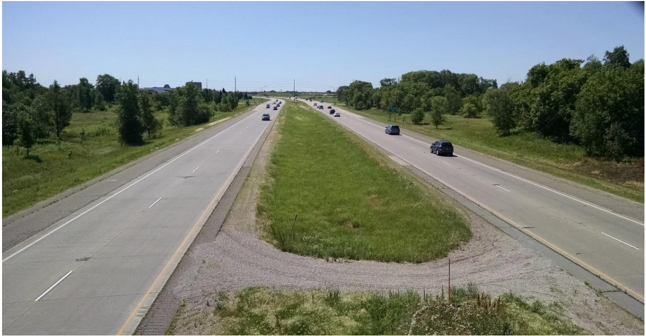
US Hwy 169 Pedestrian Bridge – From north looking south at project area.
