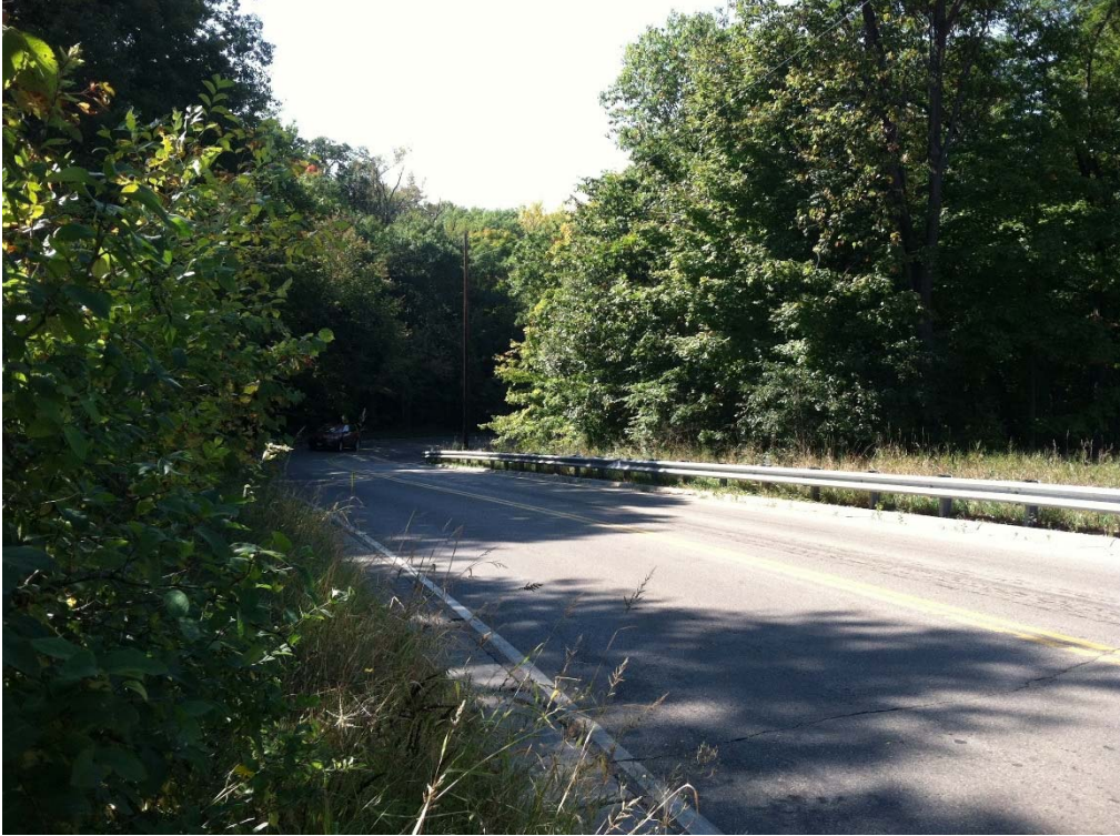
TH 101 (southbound) at Lakota Lane
