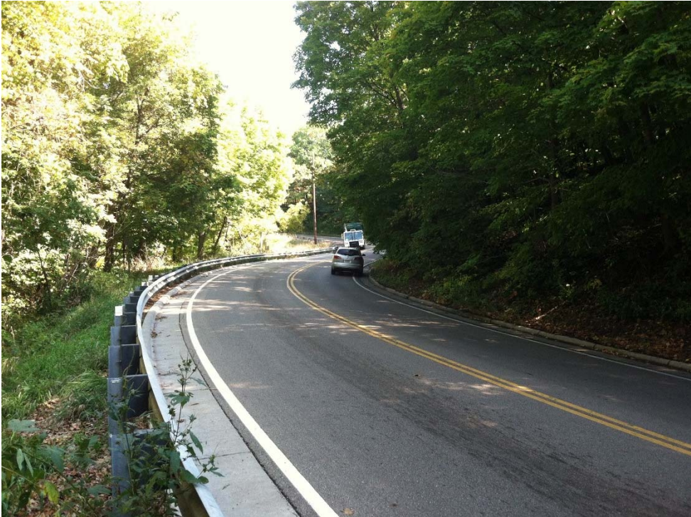
TH 101 (northbound) north of Vogelsberg Trail
