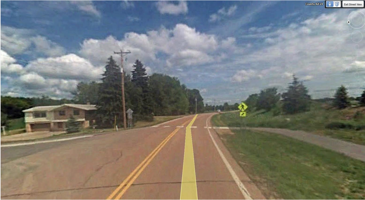
Pedestrian Crossing at Paul Ave, Looking east
