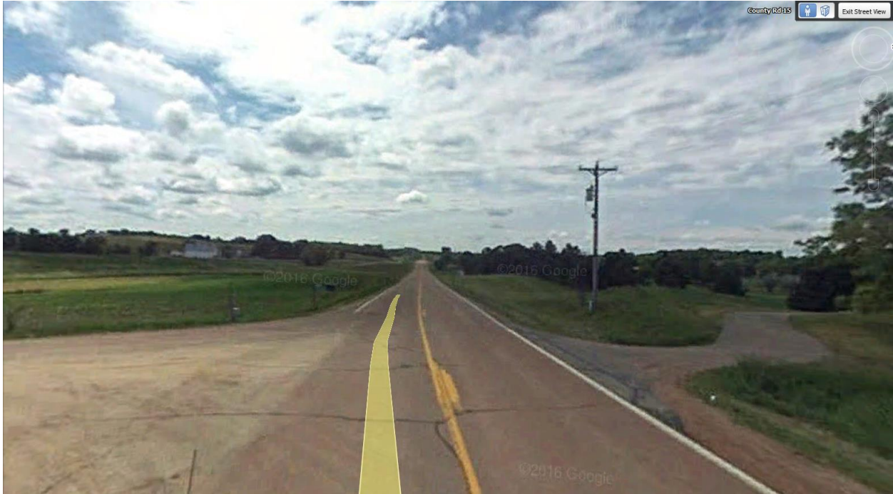
Typical residential driveway along CSAH 24
