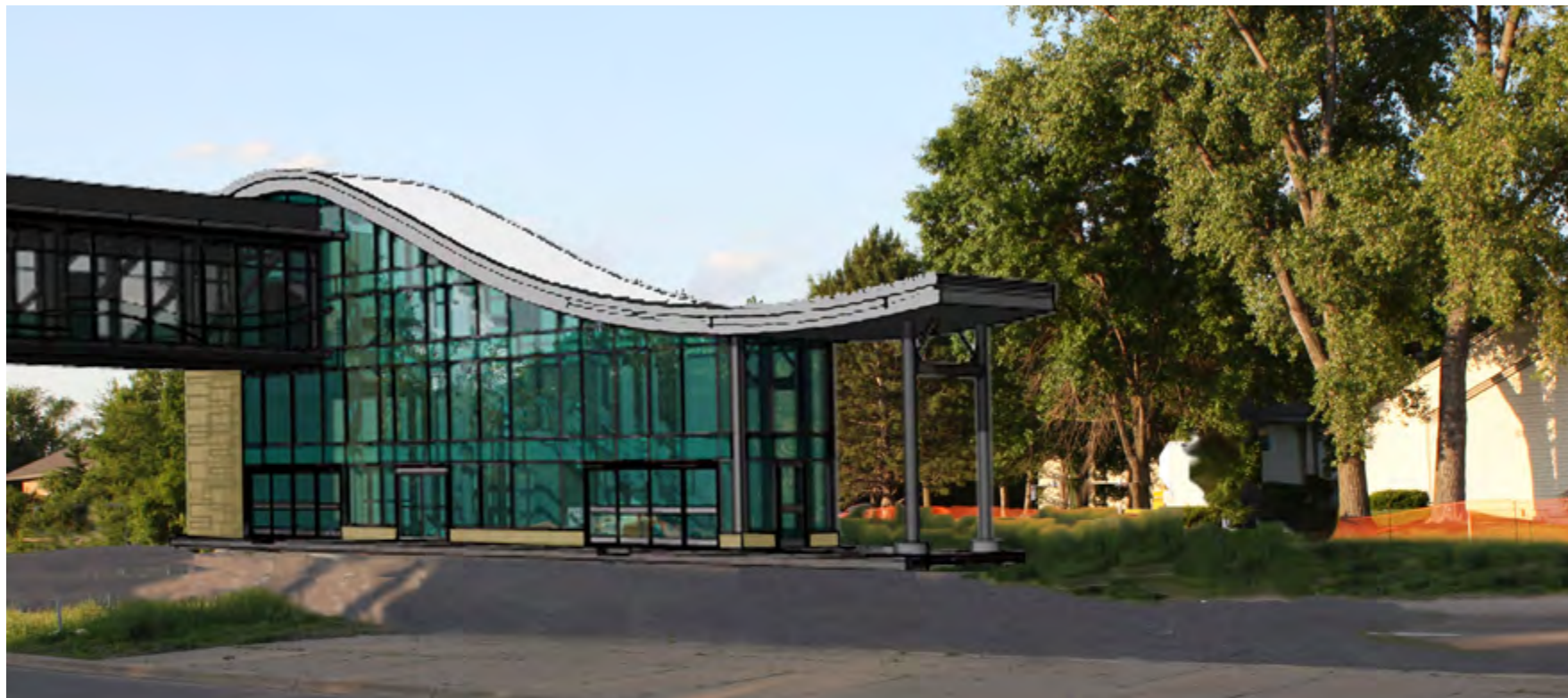
Northbound 147th Street Station Phase 2
