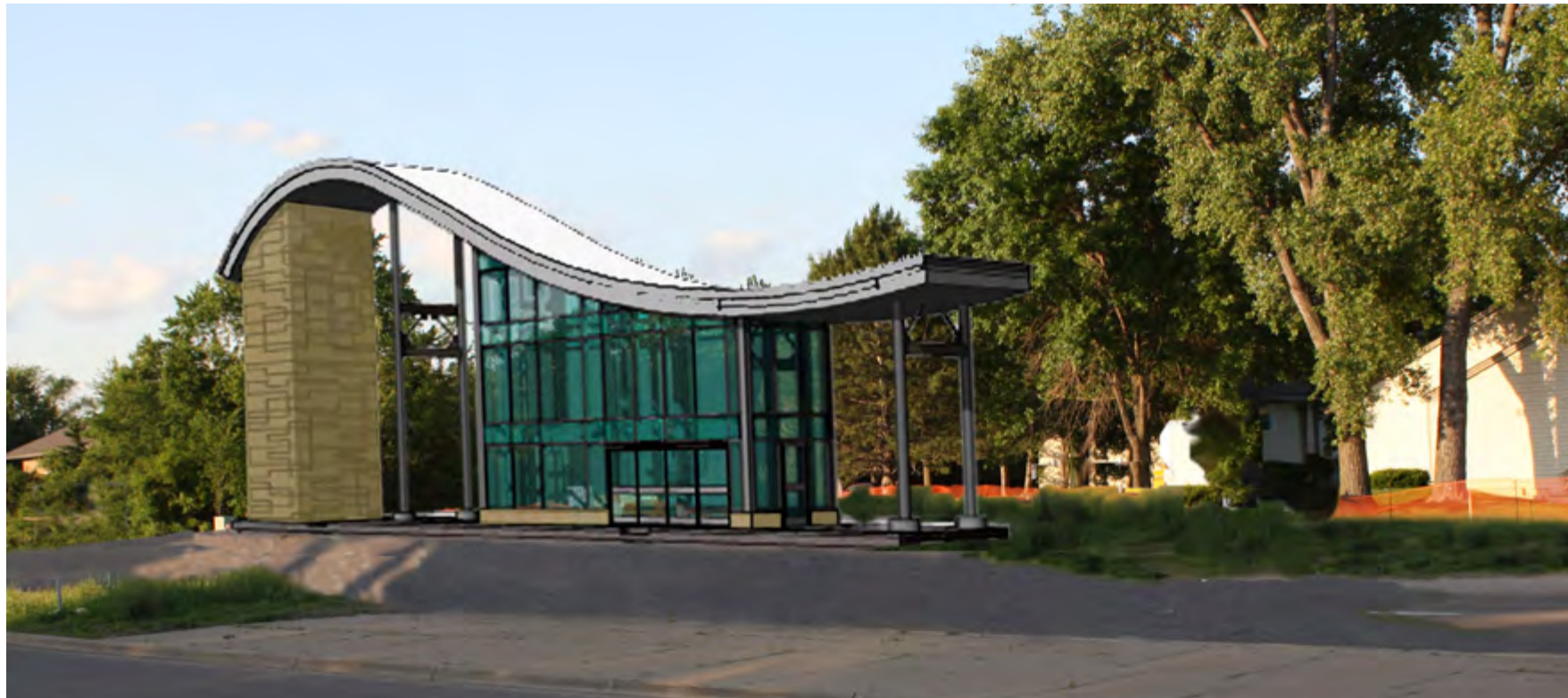
Northbound 147th Street Station Phase 1
