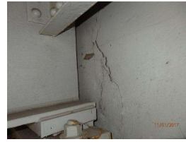
29. N Abut Backwall near center.JPG
