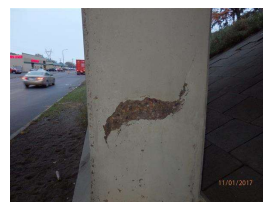
34. W side of 2nd column from the E, Pier 2.JPG
