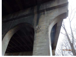
7. 2nd pier from N, E end.JPG
