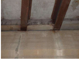
6. Diaphragm at pier 4 (1).JPG
