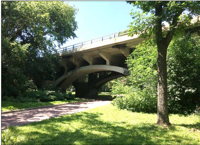
Minnehaha Parkway under Nicollet Ave. Bridge
