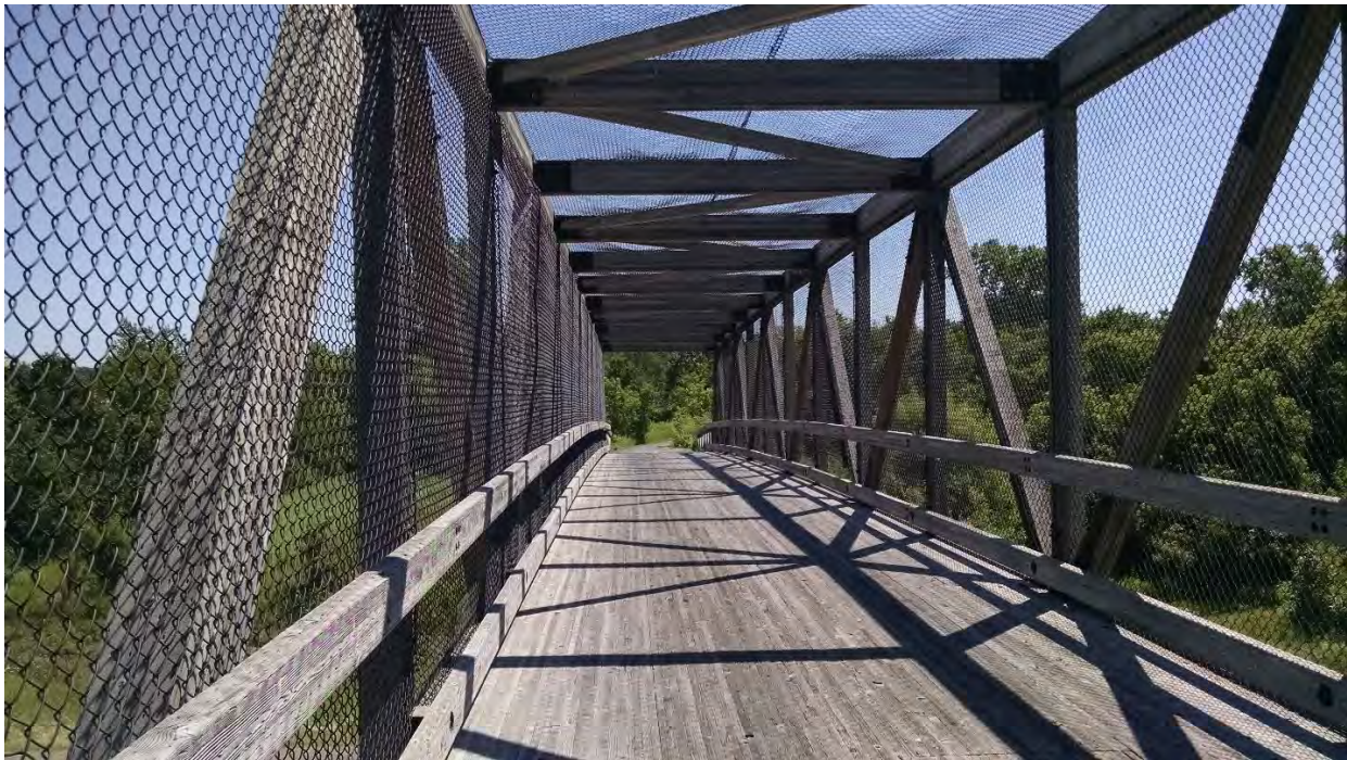
Rush Creek Trail – View from US Hwy 169 bridge west of the project area looking northeast.
