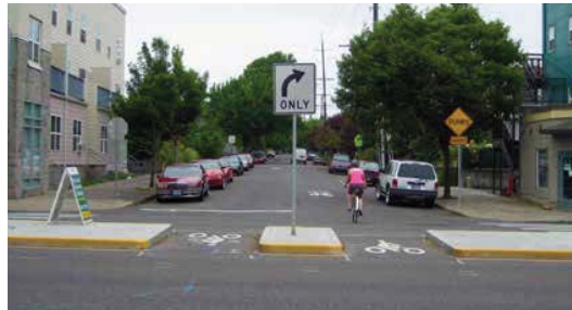
Bicycle boulevards can include treatments like this diverter that encourages drivers to take other routes.
