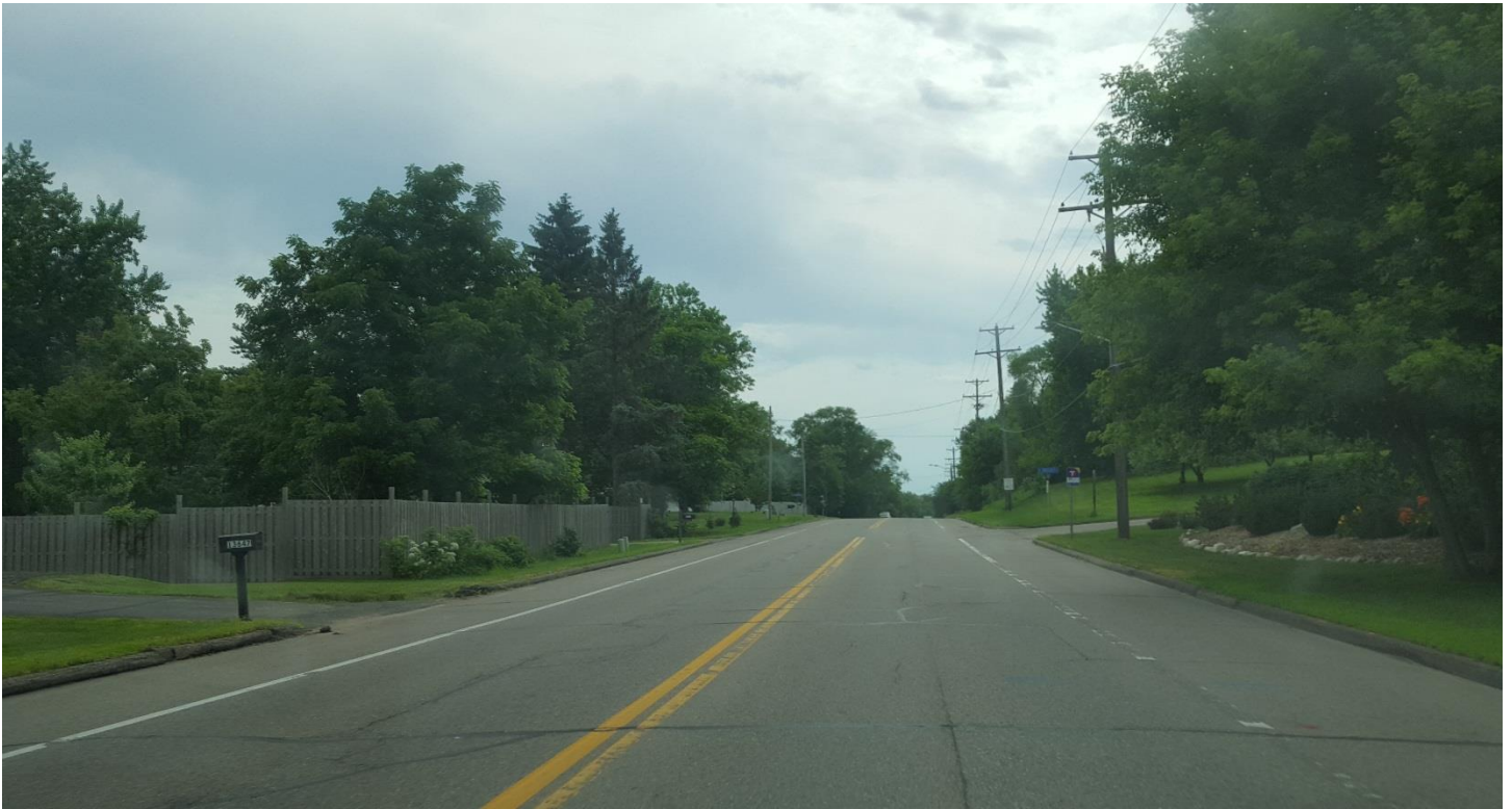
Excelsior Boulevard (CSAH 3) - looking west near Mayview Road
