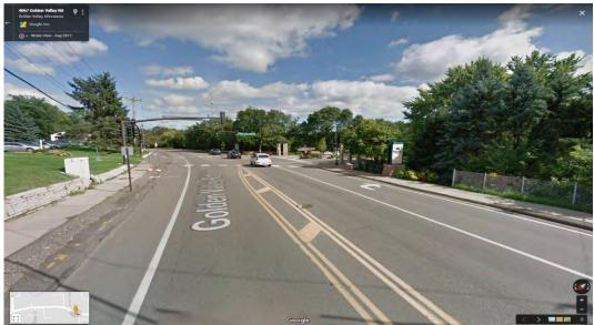
Golden Valley Road eastbound at Hidden Lakes Parkway - near Courage Kenny Center, sidewalk on north side of roadway in poor condition, sidewalk on south side narrows significantly east of this intersection. No boulevard between back of curb and sidewalk and bike lane narrows/disapears.
