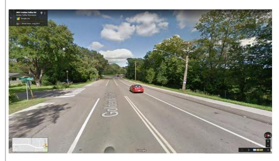
Golden Valley Road eastbound near Bonnie Lane - future Bottineau LRT connection east of this location. Theodore Wirth Park located on the south side of roadway. Sidewalk/trail not to regional trail standard, sidewalk width has been increased with pavement addition to back of bituminous curb eliminating the boulevard condition between the back of curb and sidewalk.
