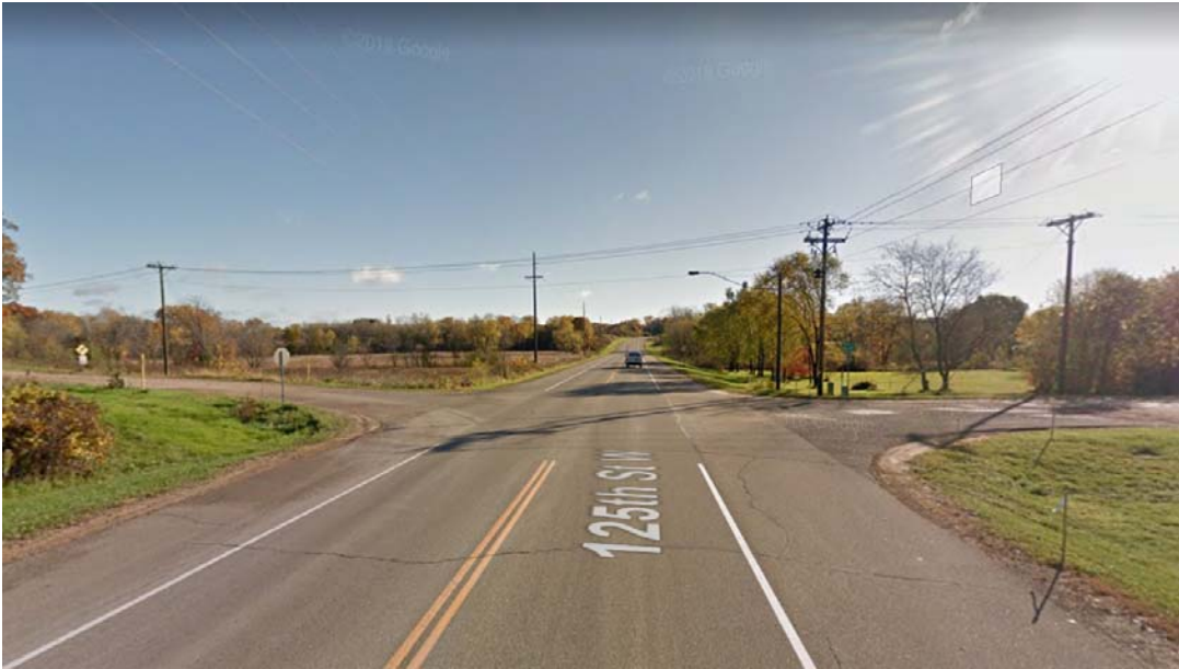
McAndrews Road (CR 38) (westbound) at Dodd Road
