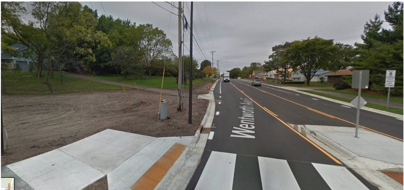
Existing Condition Photo: On Wentworth Avenue looking west.
