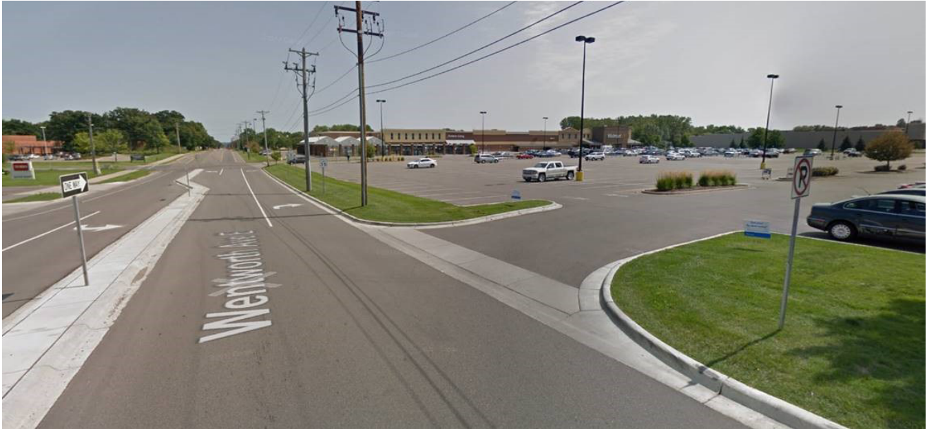
Existing Condition Photo: On Wentworth Avenue looking east toward the Wal-Mart. There is no existing sidewalk on the south side of the street.
