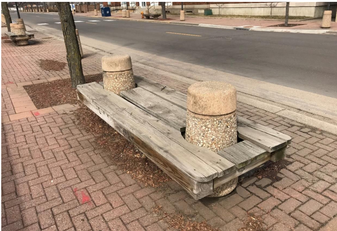
Outdated streetscape along Concord Exchange detracts from user experience and redevelopment/revitalization potential.
