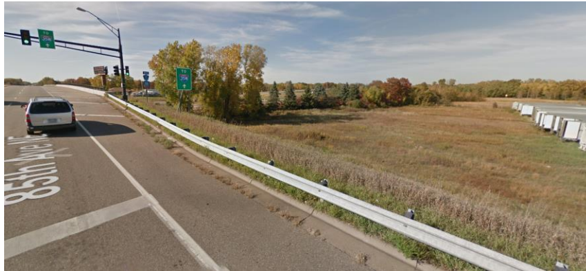
CSAH 32 LOOKING NORTHWEST (FUTURE ON-RAMP LOCATION)
