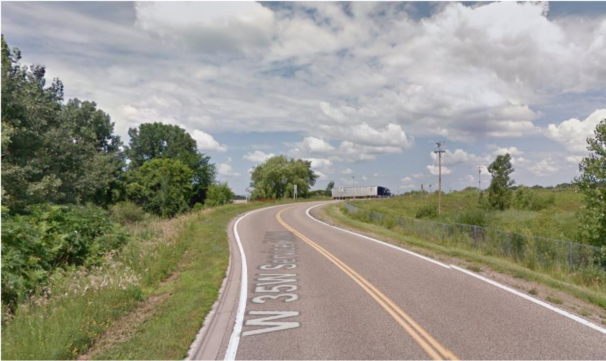
I-35W West Service Drive (northbound) at 95 th Avenue NE
