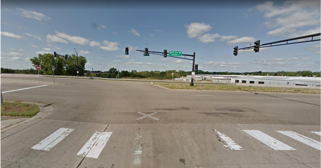
I-35W Northbound Off Ramp at CSAH 32 (Looking North)
