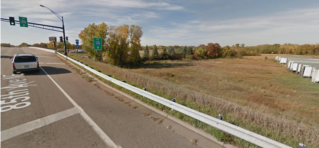
CSAH 32 (looking northwest) Future On-Ramp to I-35W
