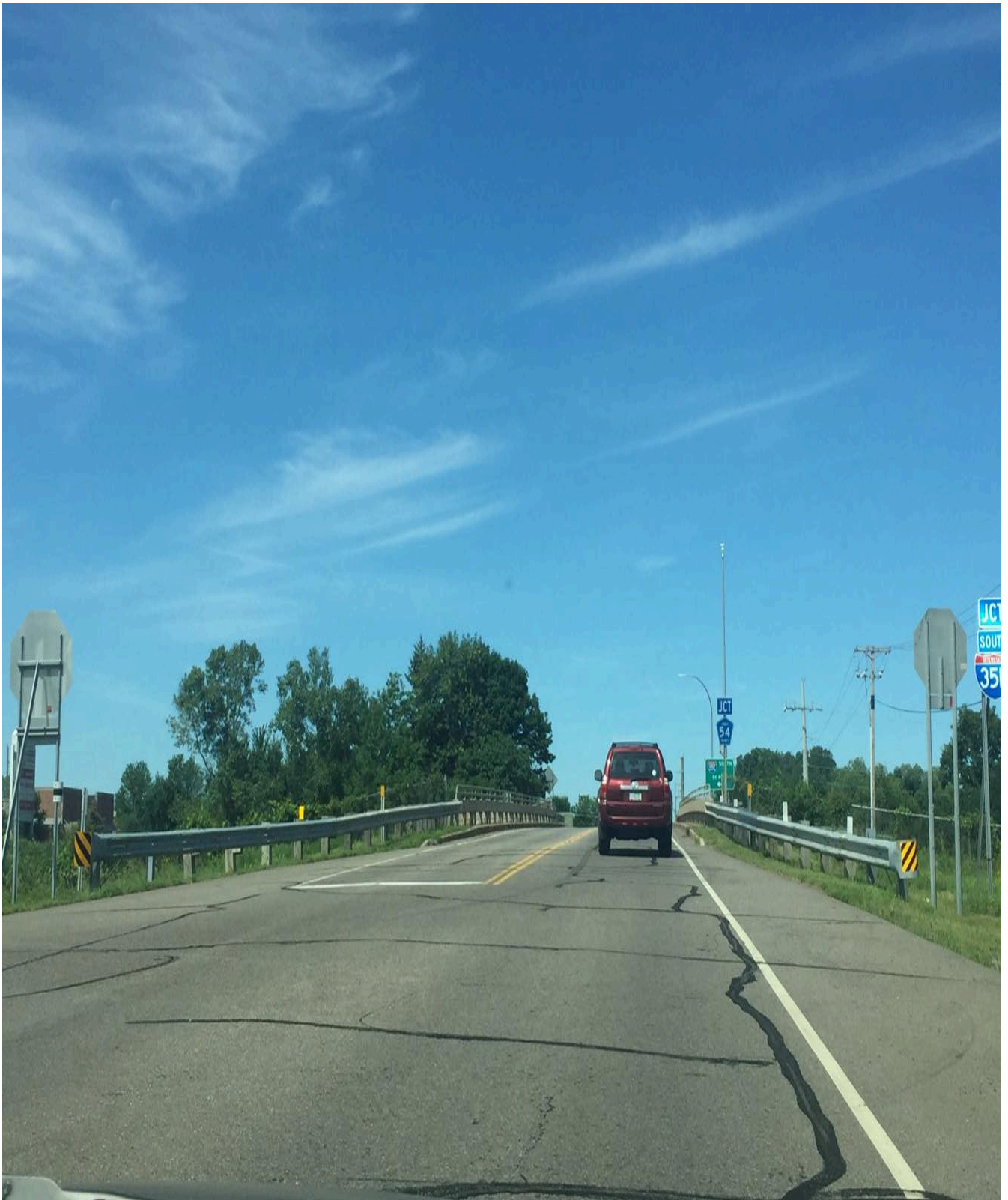
Westbound View, Showing Sight Distance Restriction
