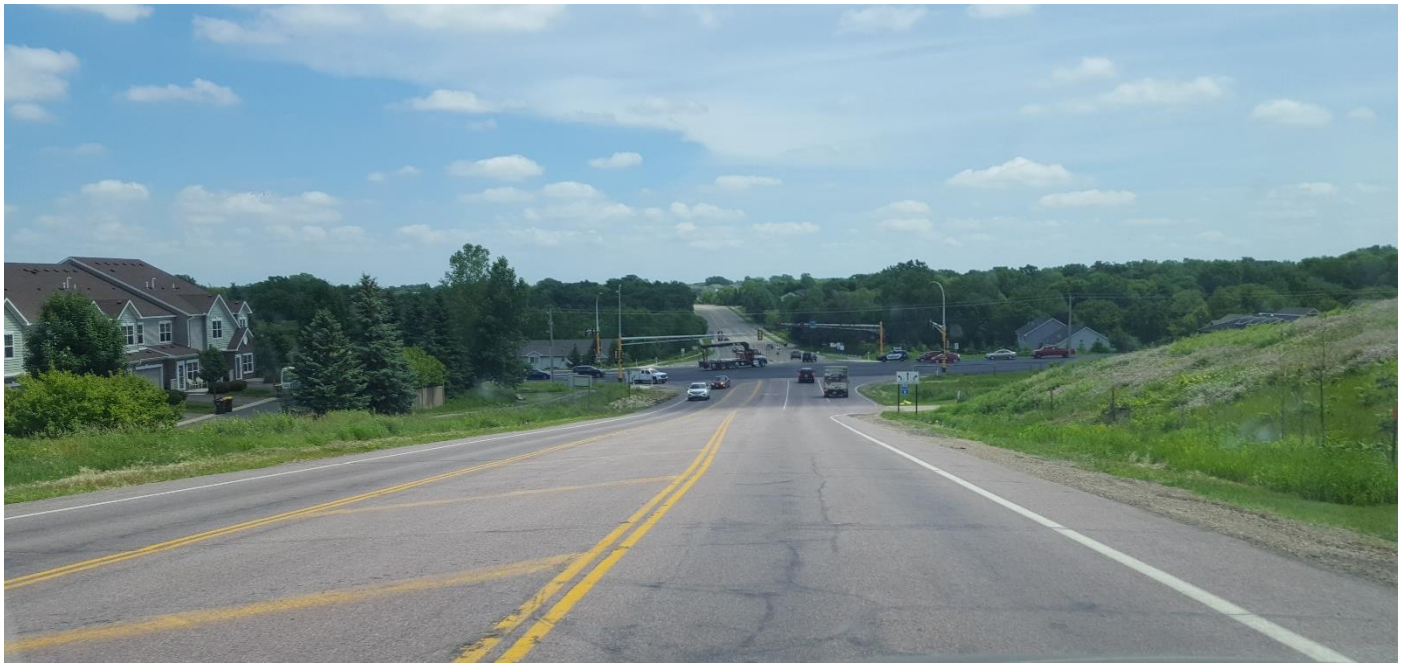
CSAH 16 – looking east towards Trunk Highway 13 intersection
