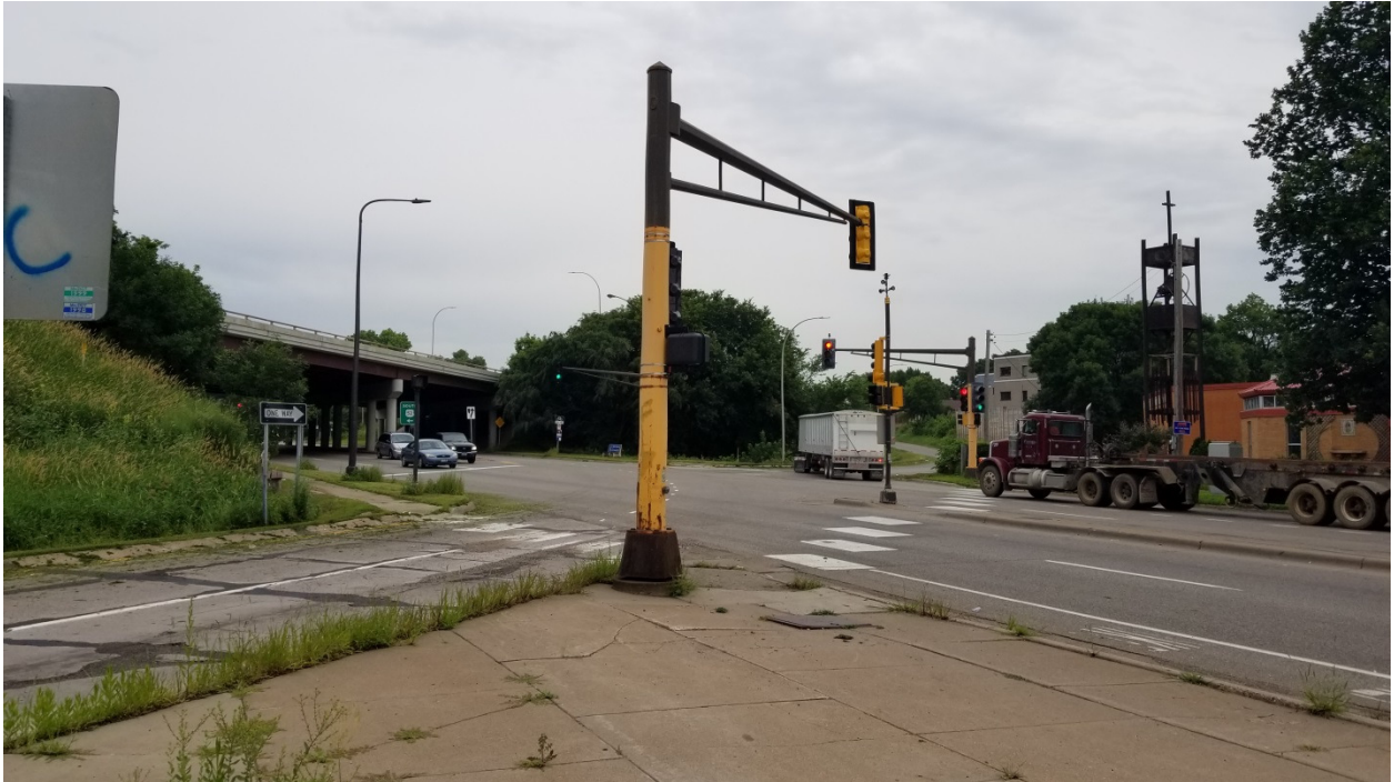
LOOKING NORTHWEST AT THE TRAFFIC SIGNAL AT CONCORD ST. (TH 156) & NORTHBOUND US 52, PROPOSED FOR RECONSTRUCTION
