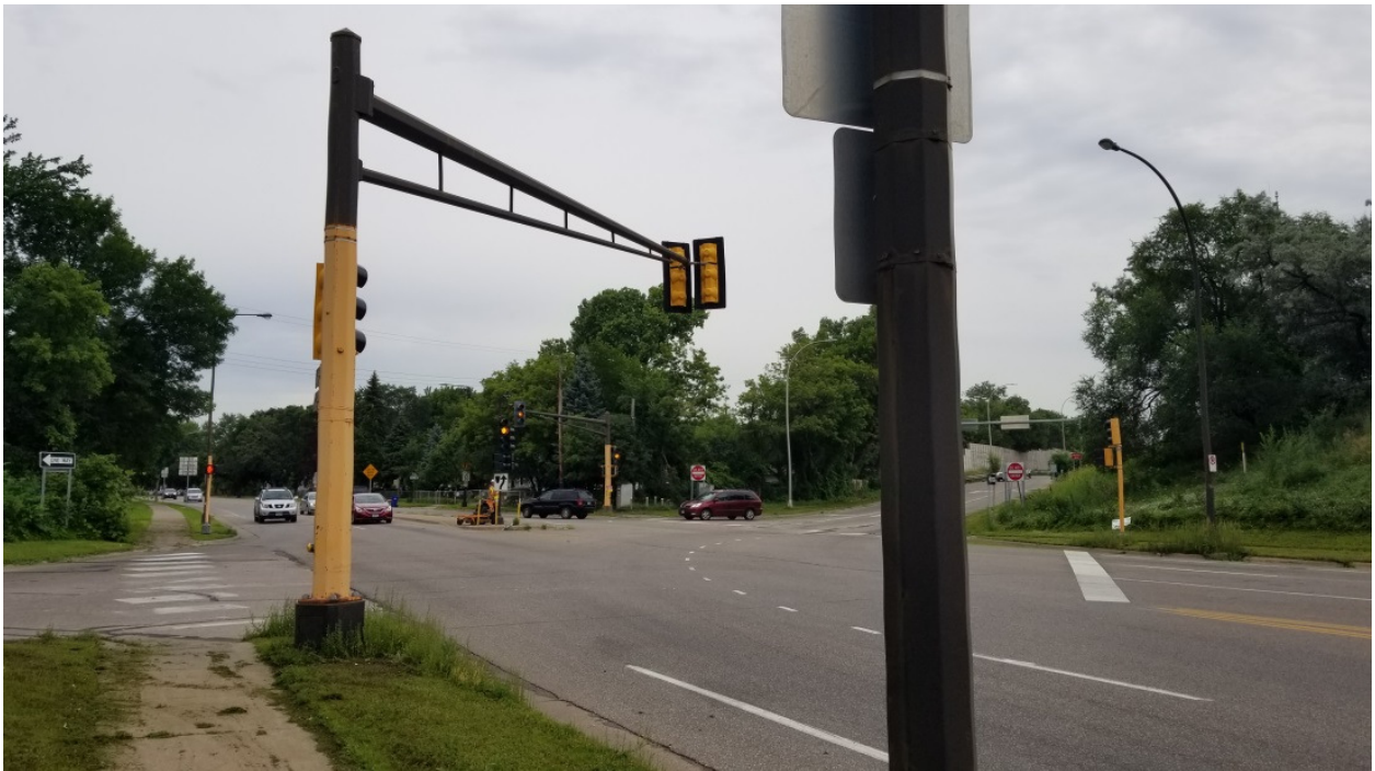
LOOKING NORTHWEST AT THE TRAFFIC SIGNAL AT CONCORD ST. (TH 156) & SOUTHBOUND US 52, PROPOSED FOR RECONSTRUCTION
