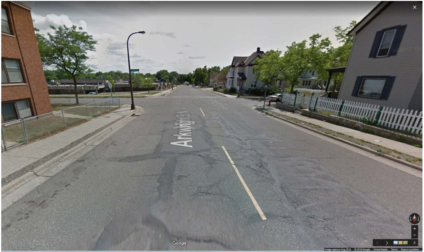
Project Components 2 & 3: Bicycle lanes and curb extensions along Arkwright Street to designate space for bicyclists, help control speeds and address wide crossings.
