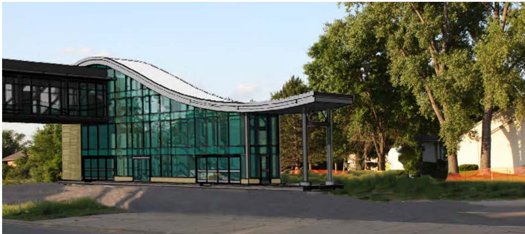
Northbound 147th Street Station Phase 2
