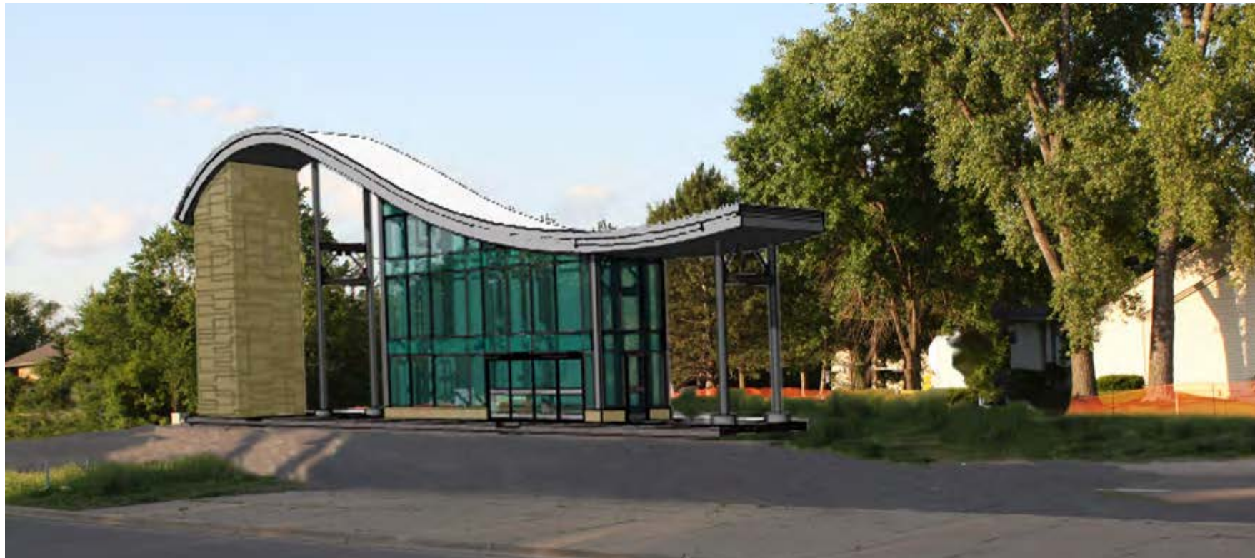
Northbound 147th Street Station Phase 1
