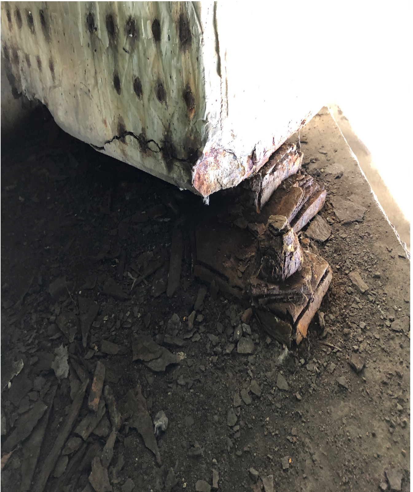
Bridge 62519 Bearing 5 condition photo
