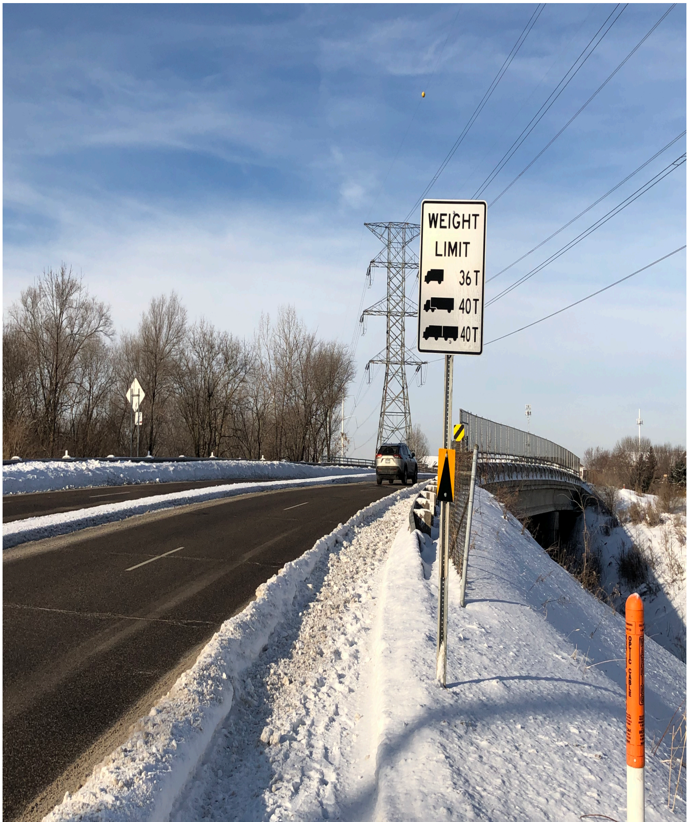
Bridge 62519 Load Posting
