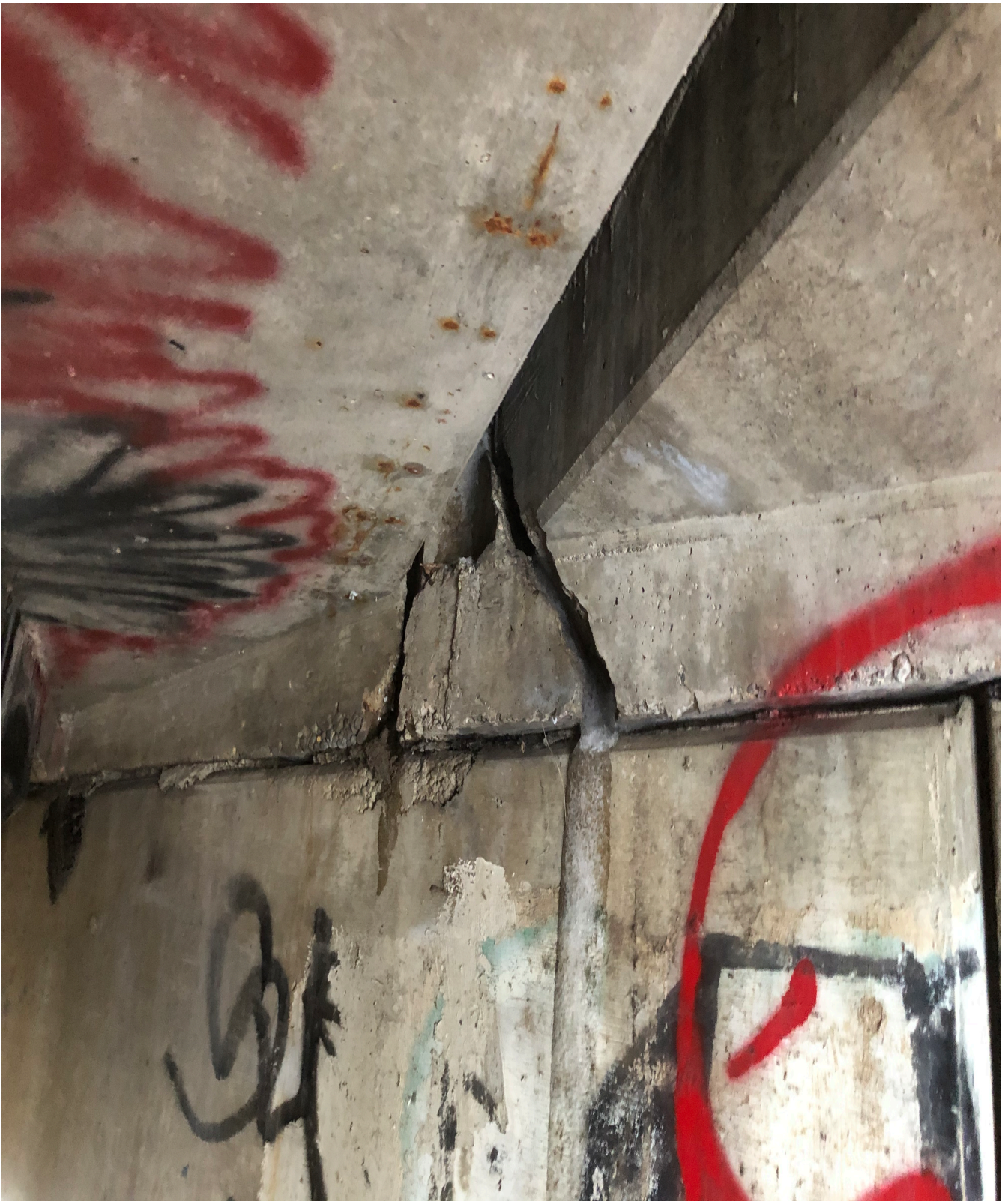
East Abutment condition photo
