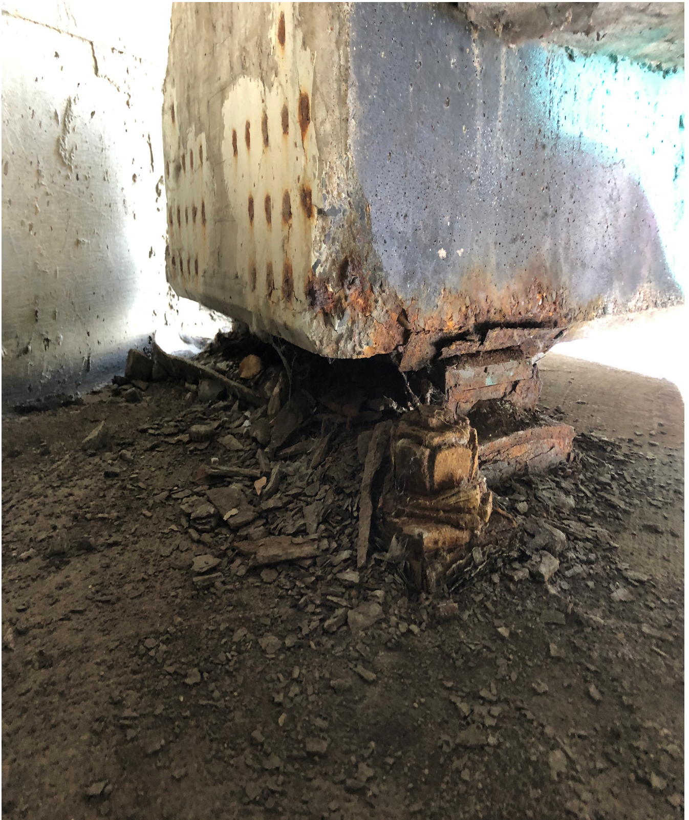
Bridge 62519 Bearing 6 condition photo
