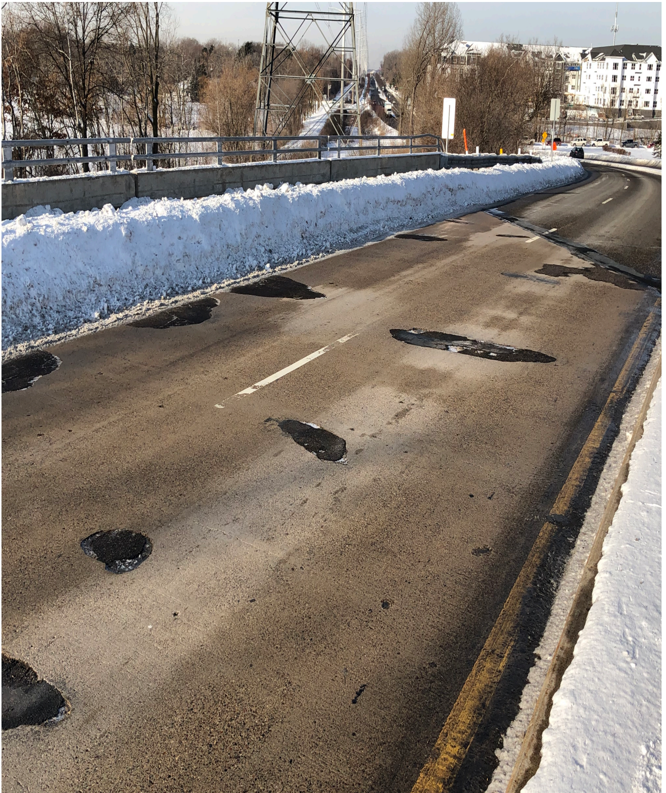
Bridge 62519 deck condition photo
