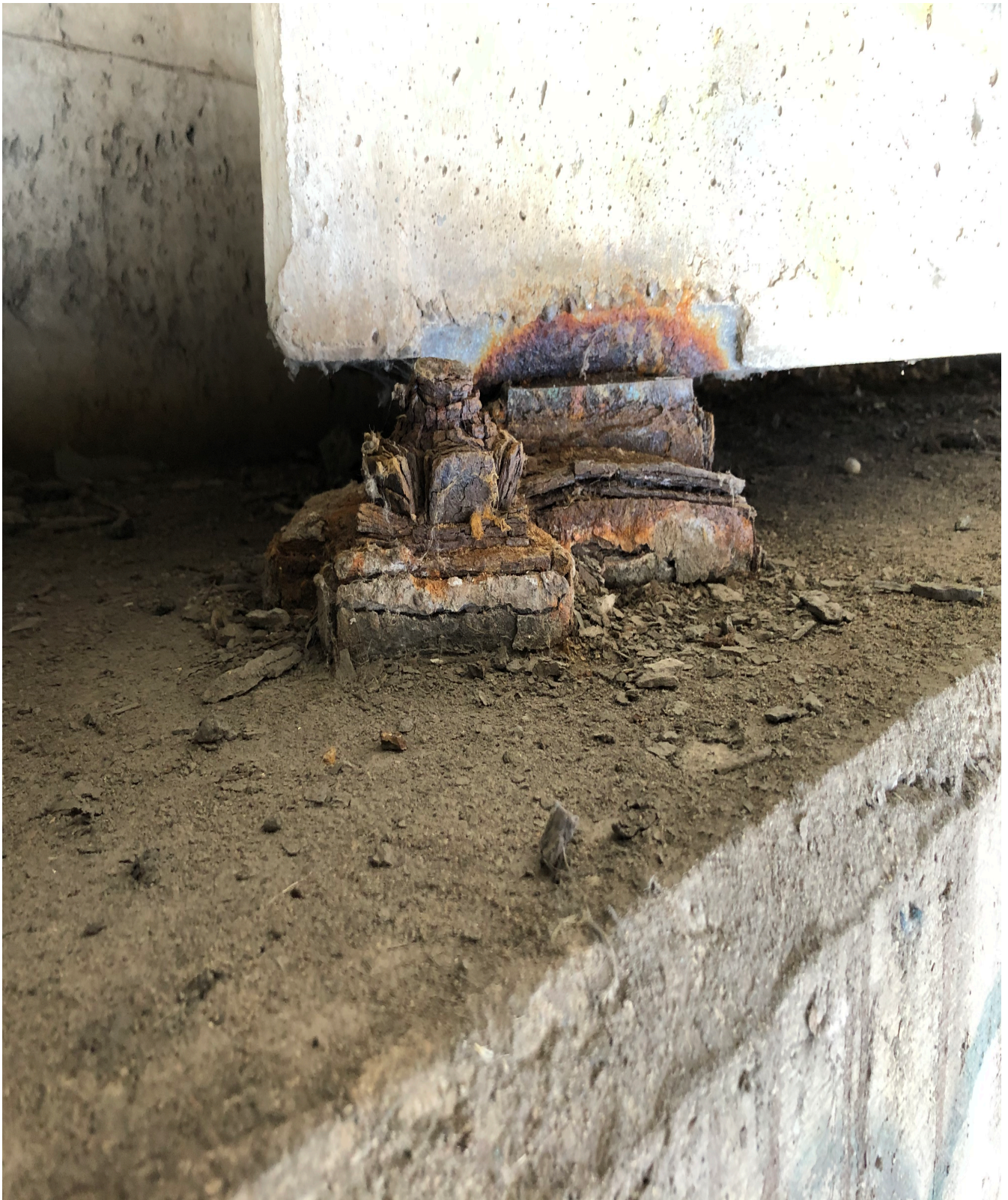
Bridge 62519 Bearing 2 condition photo
