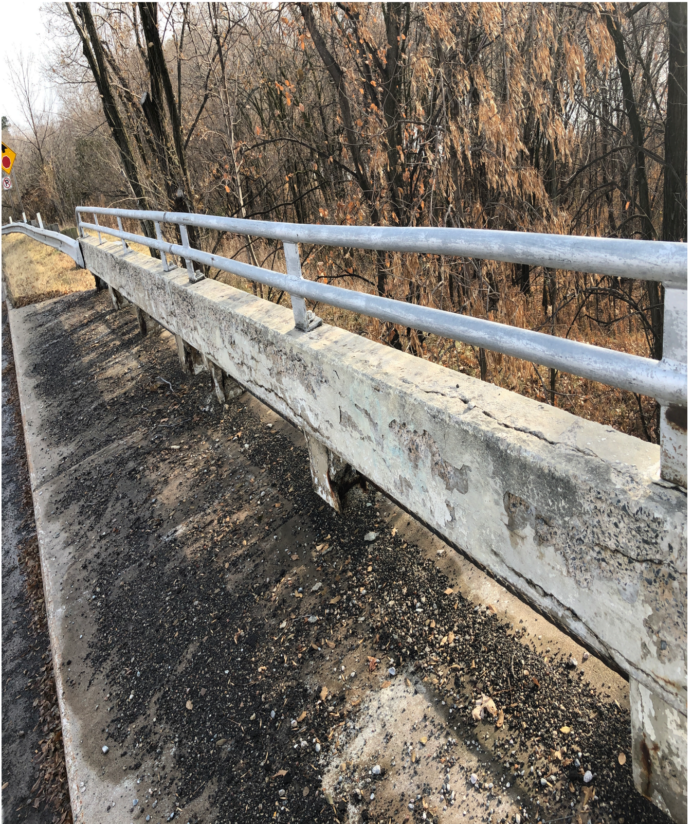
Bridge 62519 rail condition photo
