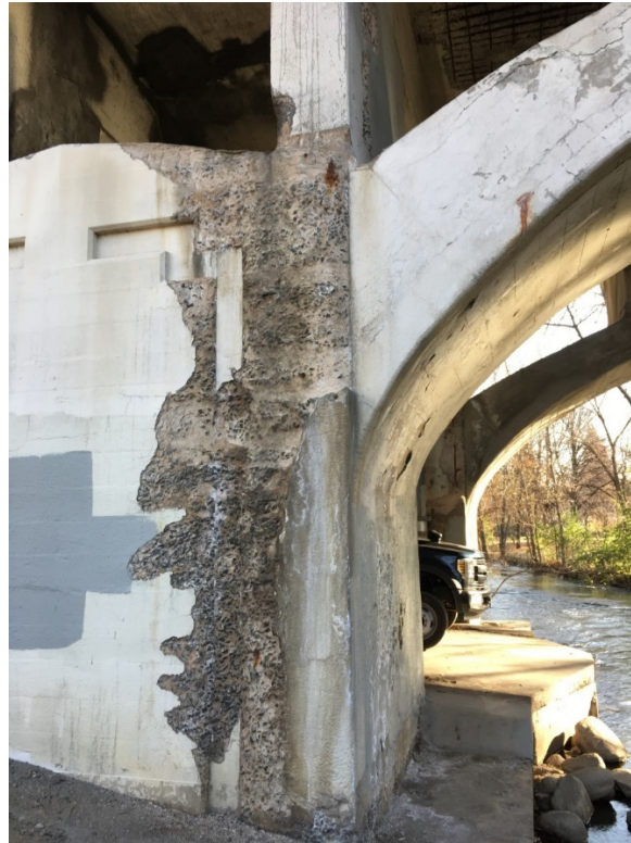
Figure 12: West Pier at Creek (2019)
