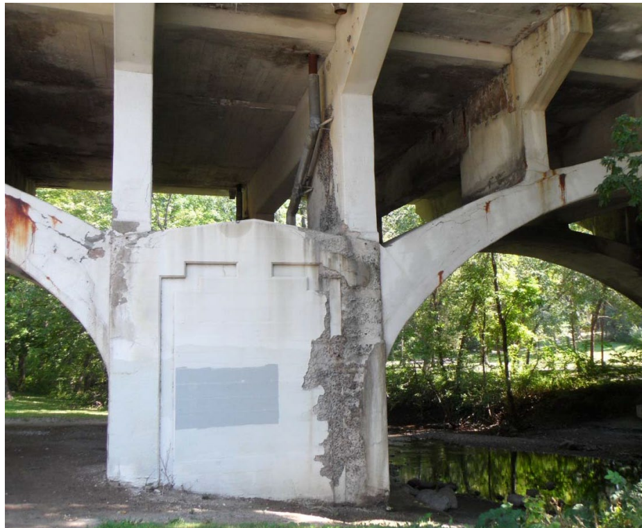
Figure 11: West Pier at Creek (2012)
