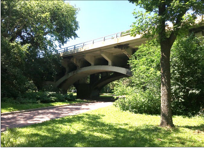
Minnehaha Parkway under Nicollet Ave. Bridge
