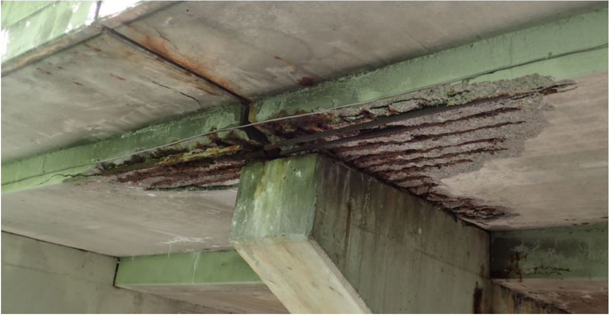
Figure 6: Deck Delamination (2019)
