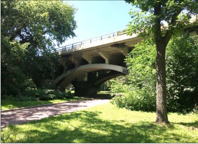
Minnehaha Parkway under Nicollet Ave. Bridge
