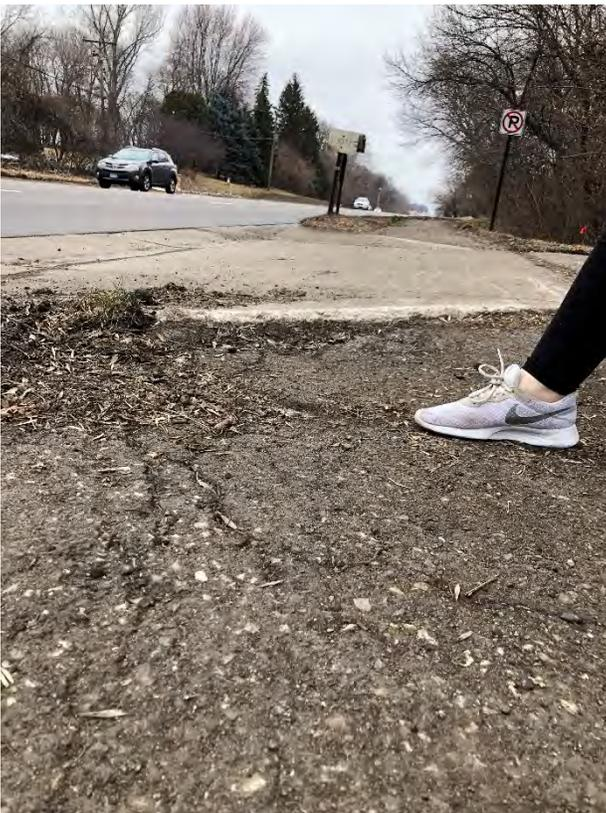
Fig 7. W 102<sup>nd</sup> to Old Shakopee Road, East side – Example of ADA concerns with holes and driveway transitions
