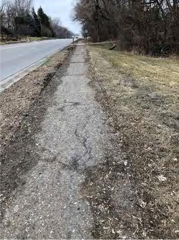
Fig 6. W 102<sup>nd</sup> to Old Shakopee Road, East side –Example of deteriorated pavement and subgrade, narrow boulevard
