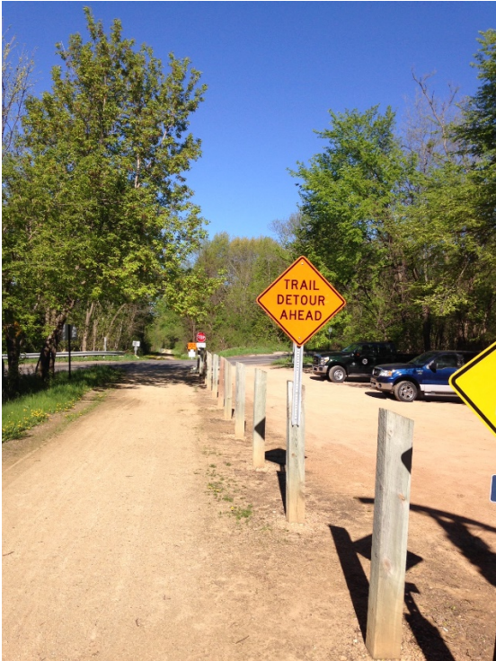
Figures 1-3 –Trail closures and detour due to 2014 landslide damage
