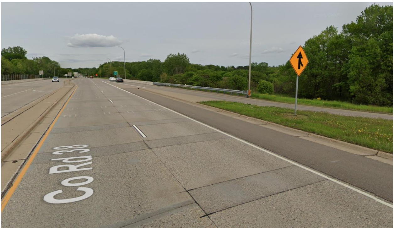
Existing Conditions: CSAH 38 westbound at Cedar Avenue (TH77) intersection, with merging onramp; no shoulder facilities.
