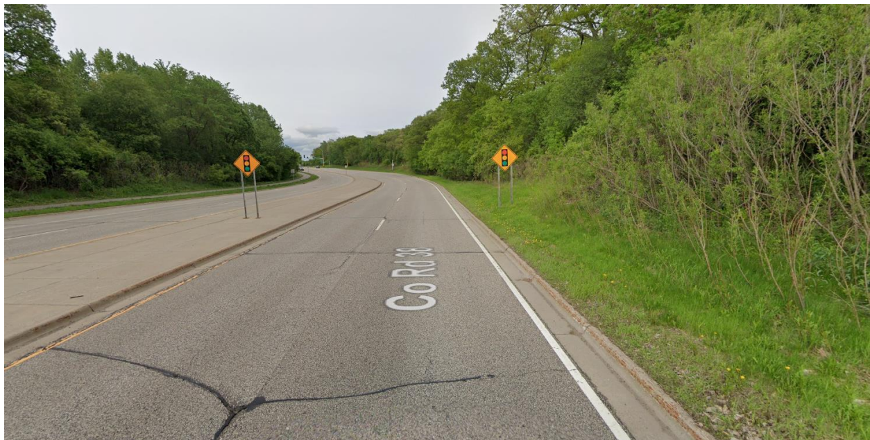
Existing Conditions: CSAH 38 eastbound, approaching Pennock Avenue. No shoulder facilities exist here for cyclists/pedestrians
