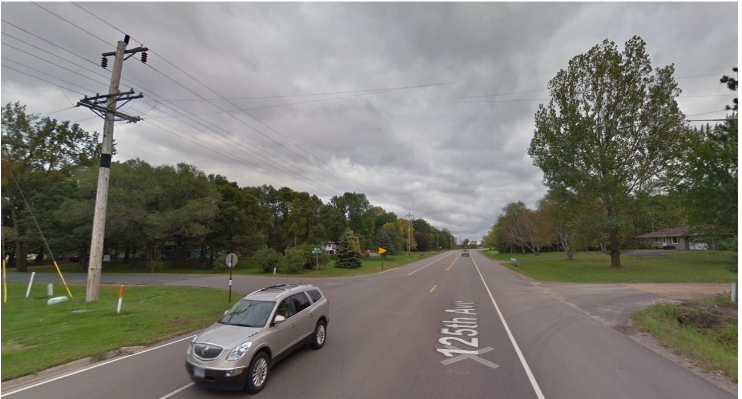
Intersection of Main Street (CSAH 14) and West Rondeau Lake Drive; wide shoulder with no barriers between high speed traffic and pedestrians and bicyclists – facing east
