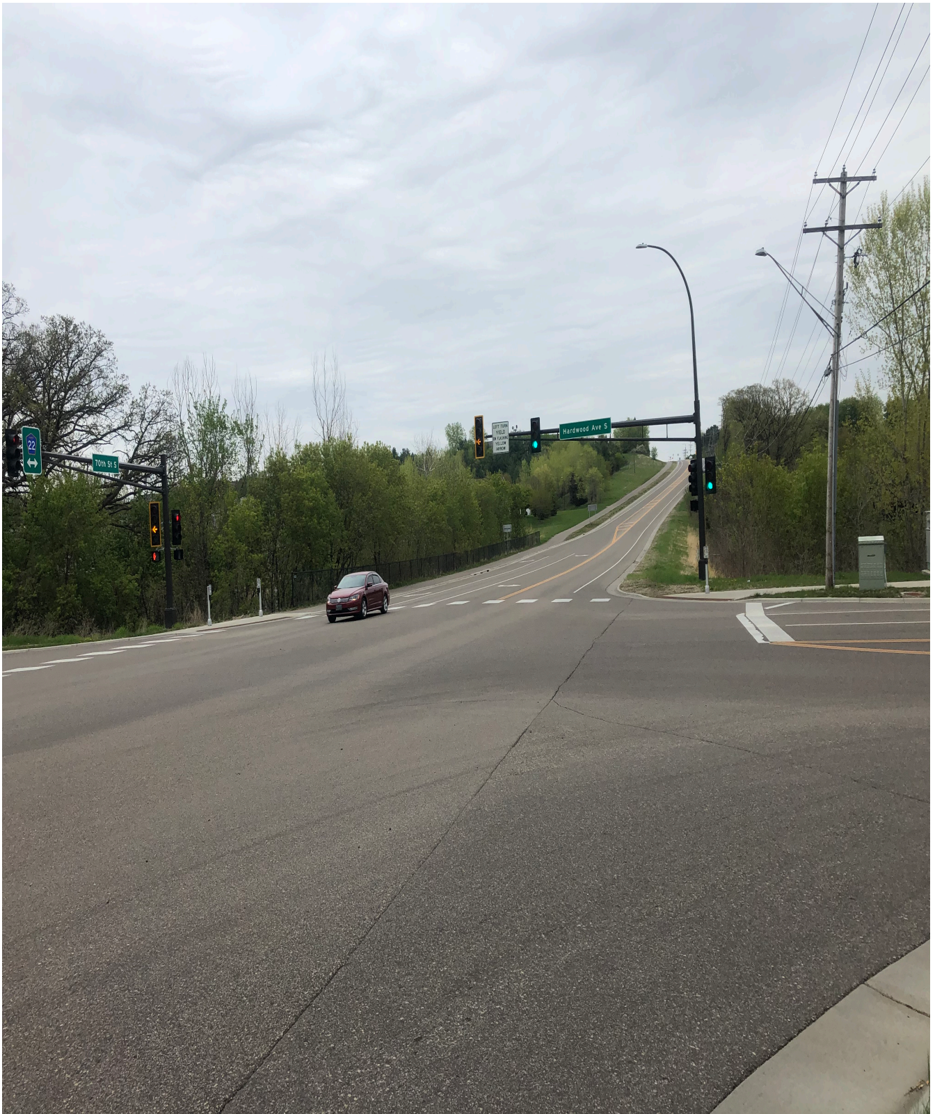
Photo of existing site_CSAH 22 Underpass
