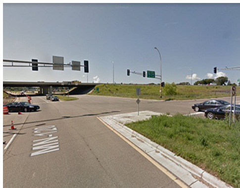
Figure 41. Century Avenue and I-94 Intersection
