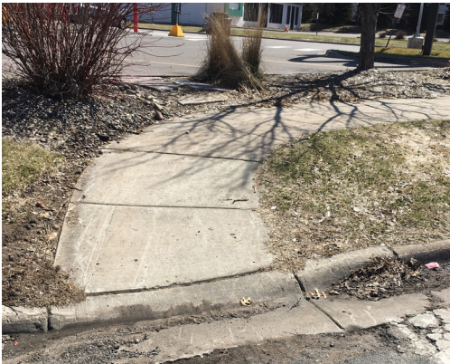
Project Location #18, example of existing pedestrian curb ramp in need of replacement to comply with ADA standards
