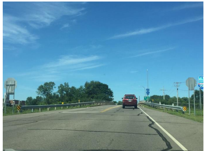
Westbound County Road J east of I-35E West Ramp
