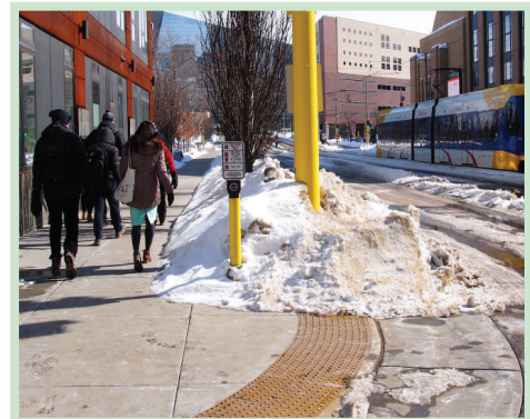
Representative ADA-compliant pedestrian curb ramps and Accessible Pedestrian Signals (APS)
