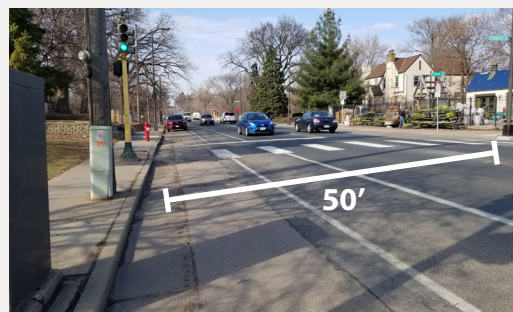
Typical existing cross section with a narrow sidewalk located at the back of curb, parking lanes, on-street bike lanes and two vehicle lanes.
