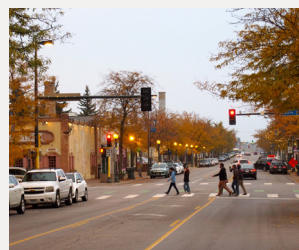
Upgraded Traffic Signals and Enhanced Lighting
