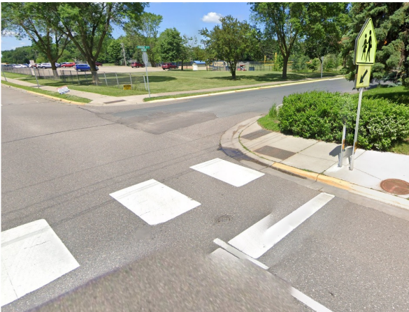
Pavement rehabilitation and new crosswalk on the north leg of the Johnson Street intersection
