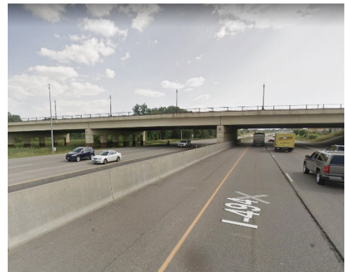
Figure 13. I-494 Station Access Barrier
