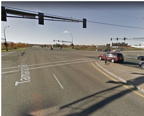
Figure 6. Tamarack Road Barrier
