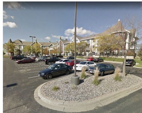
Figure 18. Guider Drive Apartments
