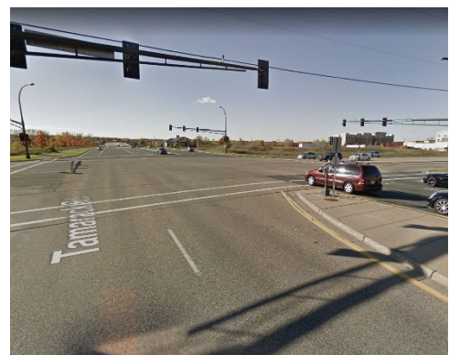
Figure 14. Tamarack Station Access Barrier
