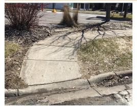
Project Location #18, example of existing pedestrian curb ramp in need of replacement to comply with ADA standards
