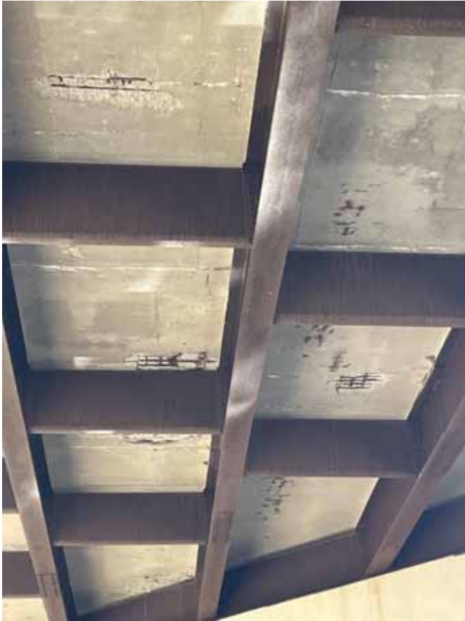
Concrete spalling and cracking as shown from the Minnesota River Bluffs LRT Regional Trail below CSAH 1.
