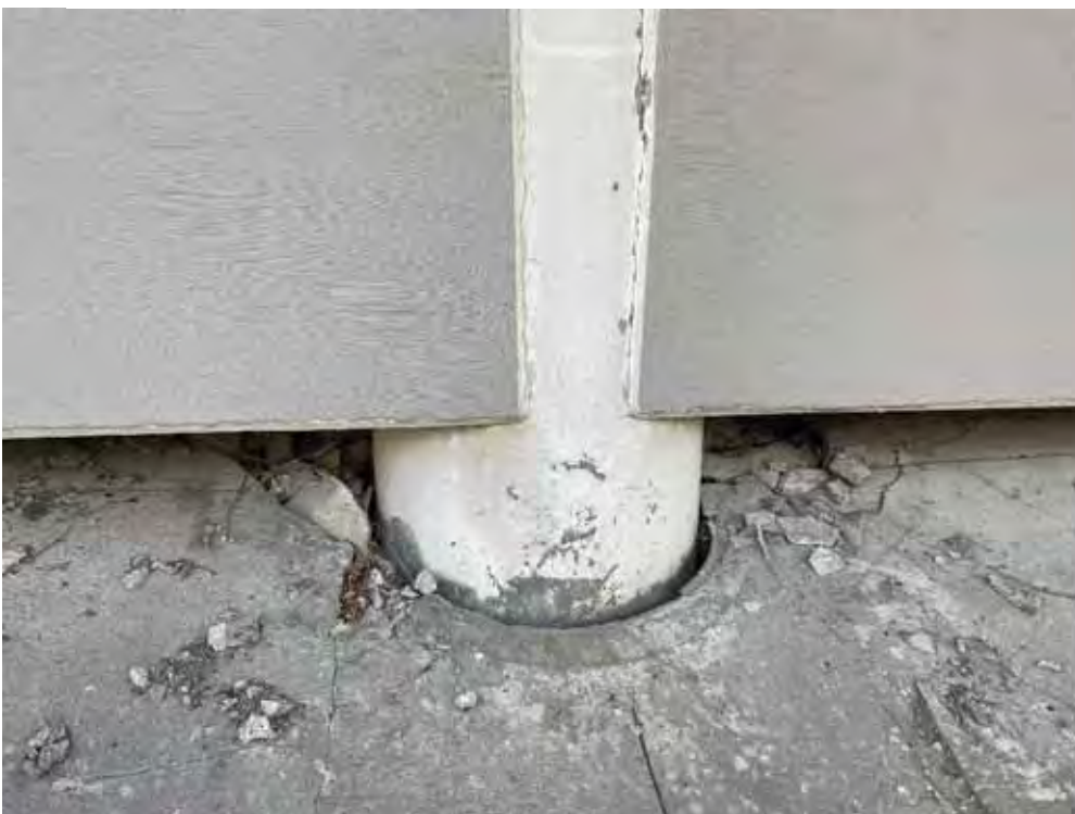
Concrete spalling and cracking as shown from the Minnesota River Bluffs LRT Regional Trail below CSAH 1.
