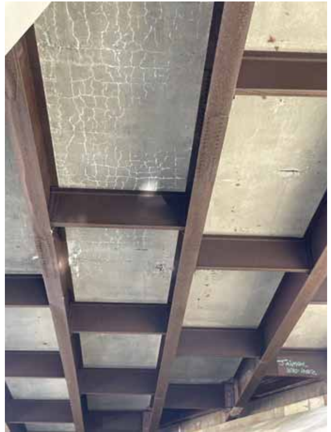
Concrete spalling and cracking as shown from the Minnesota River Bluffs LRT Regional Trail below CSAH 1.
