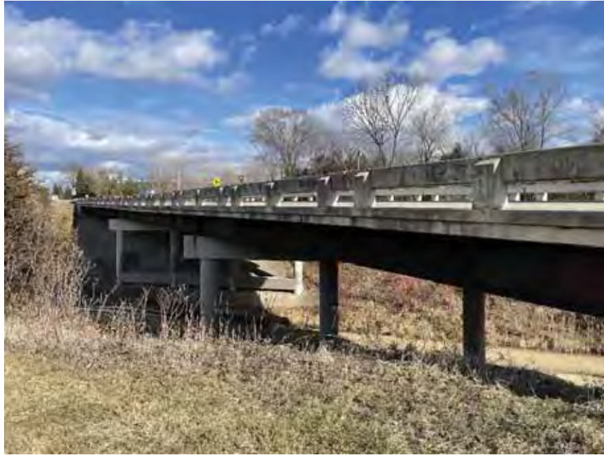
Side profile of existing bridge
