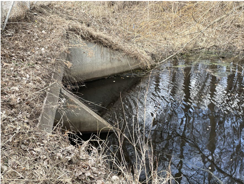
North culvert intake.
