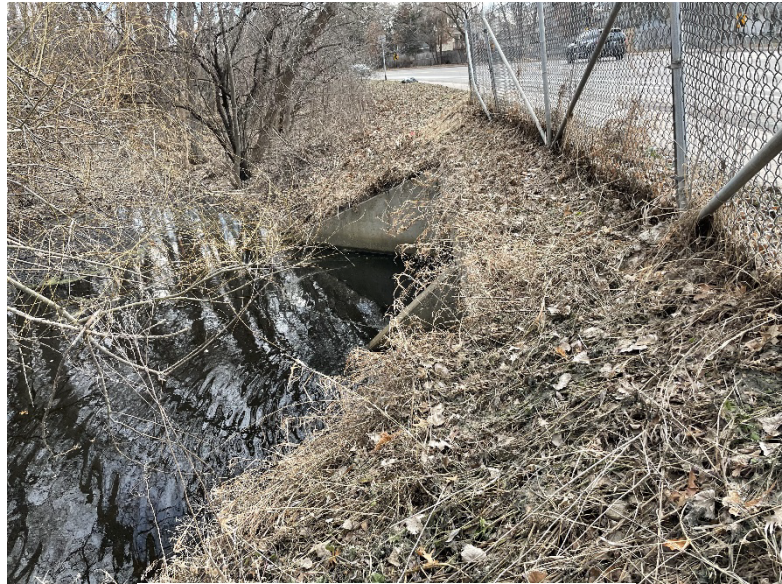
South culvert intake.
