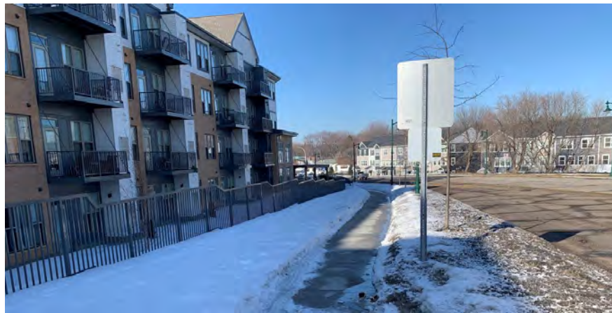
Existing Sidewalk Approaching Bridge From South
