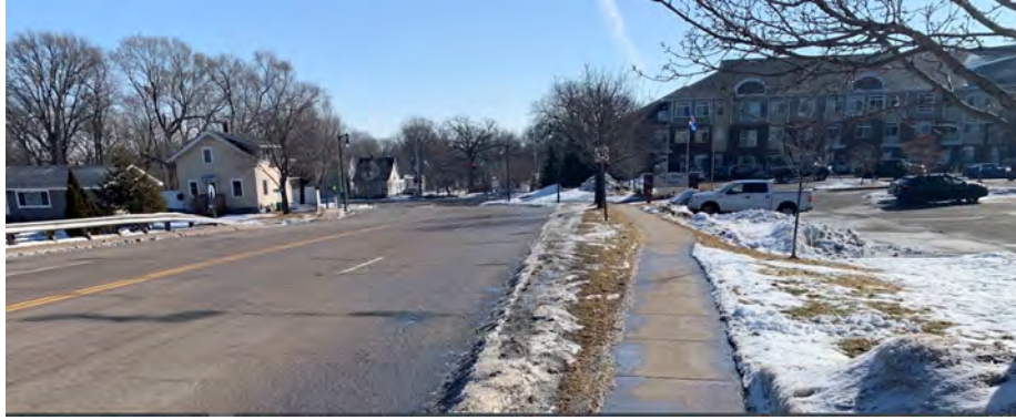
Existing Sidewalk Approaching Bridge From North
