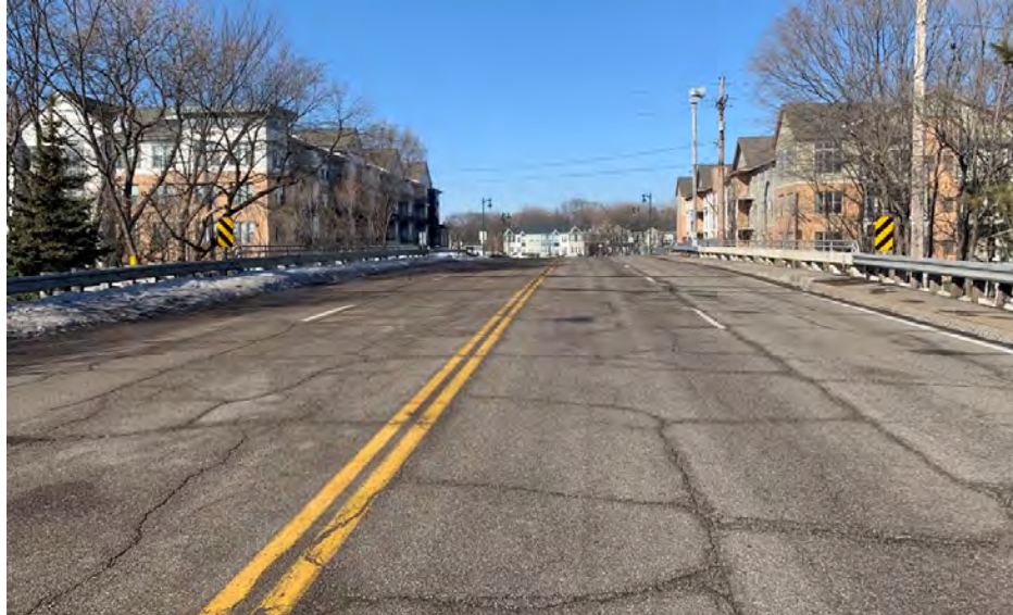
Existing Bridge Looking South
