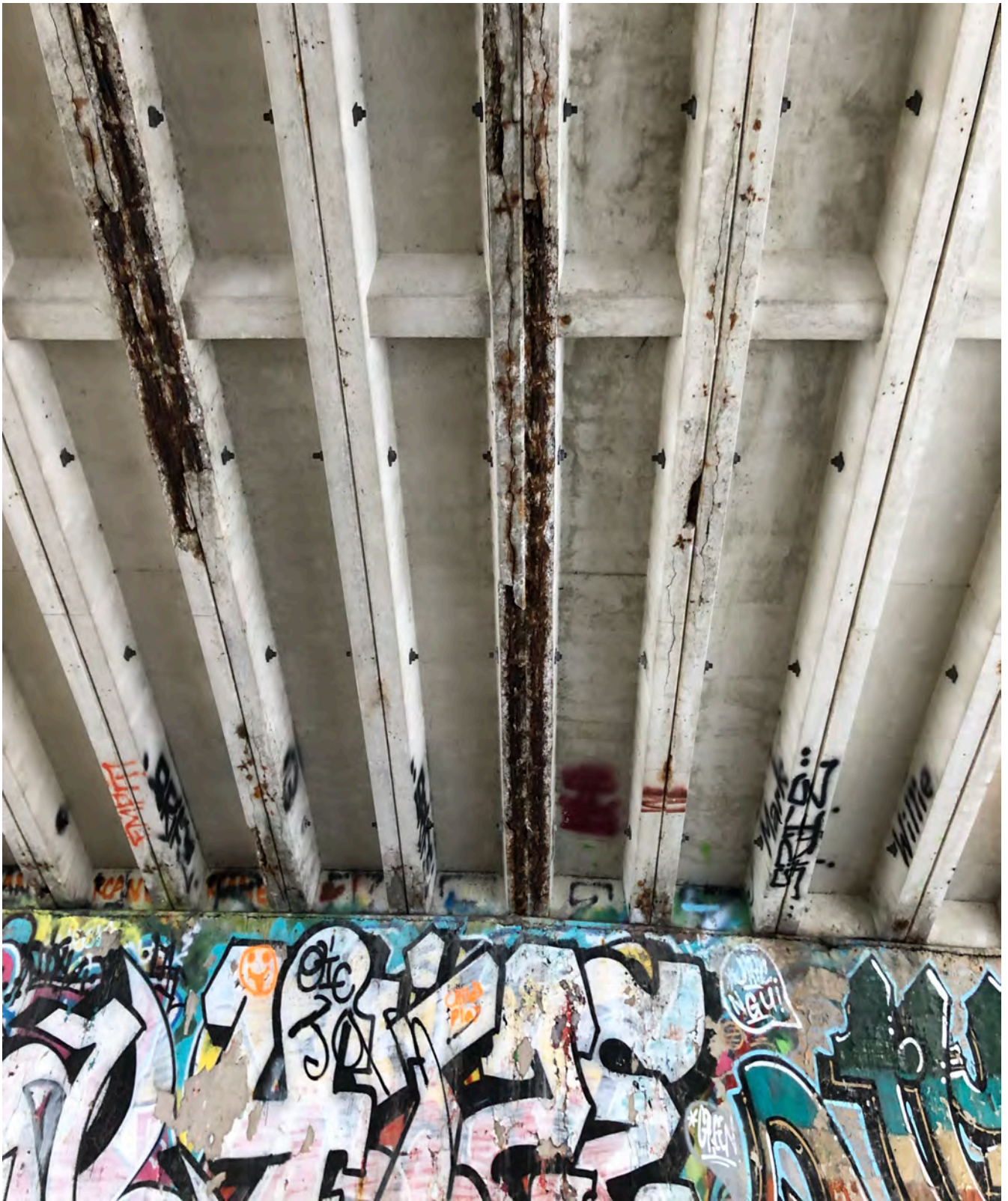
Bridge 4533 beam condition
