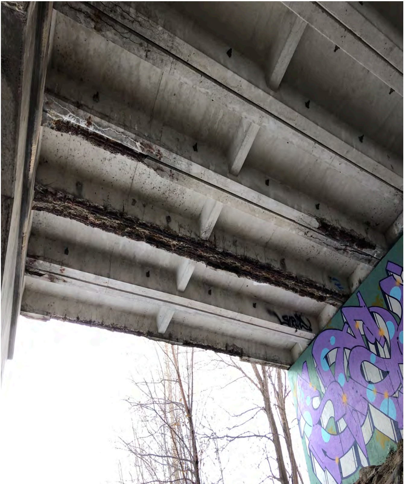
Bridge 4533 beam condition
