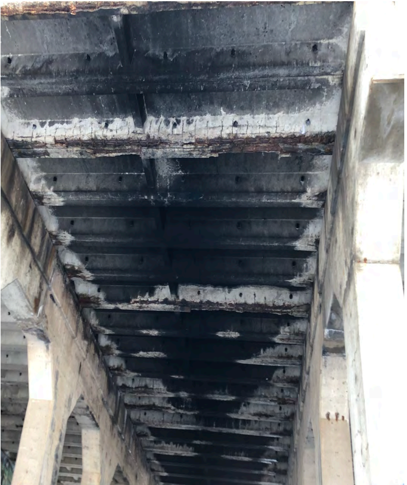
Bridge 4533- beam condition
