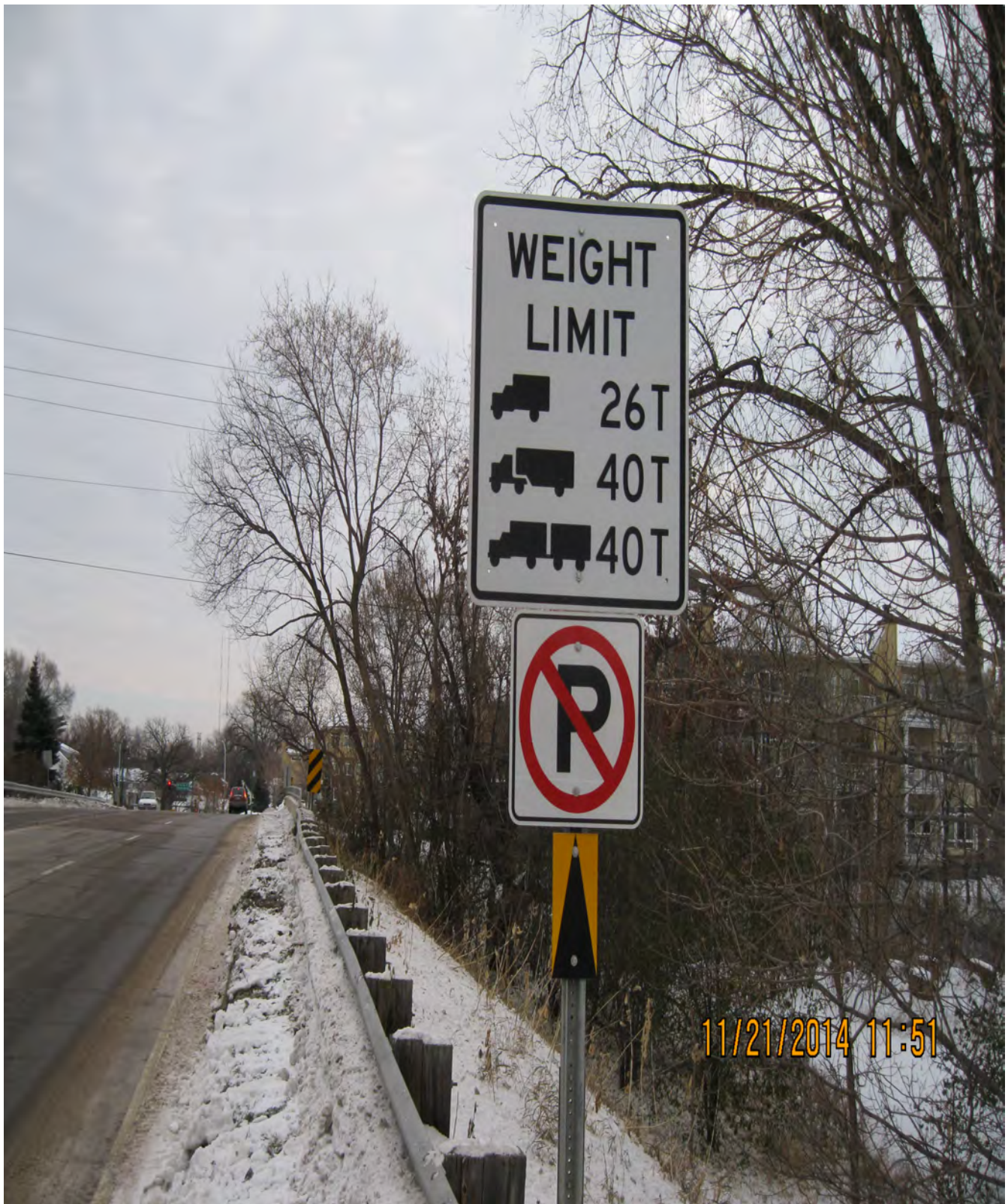
Bridge 4533 Load Limits
