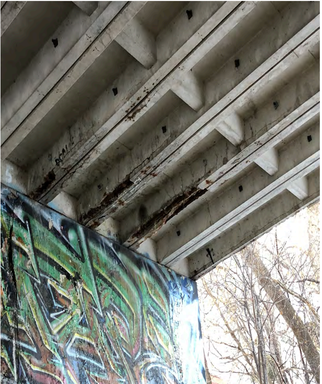
Bridge 4533- beam condition
