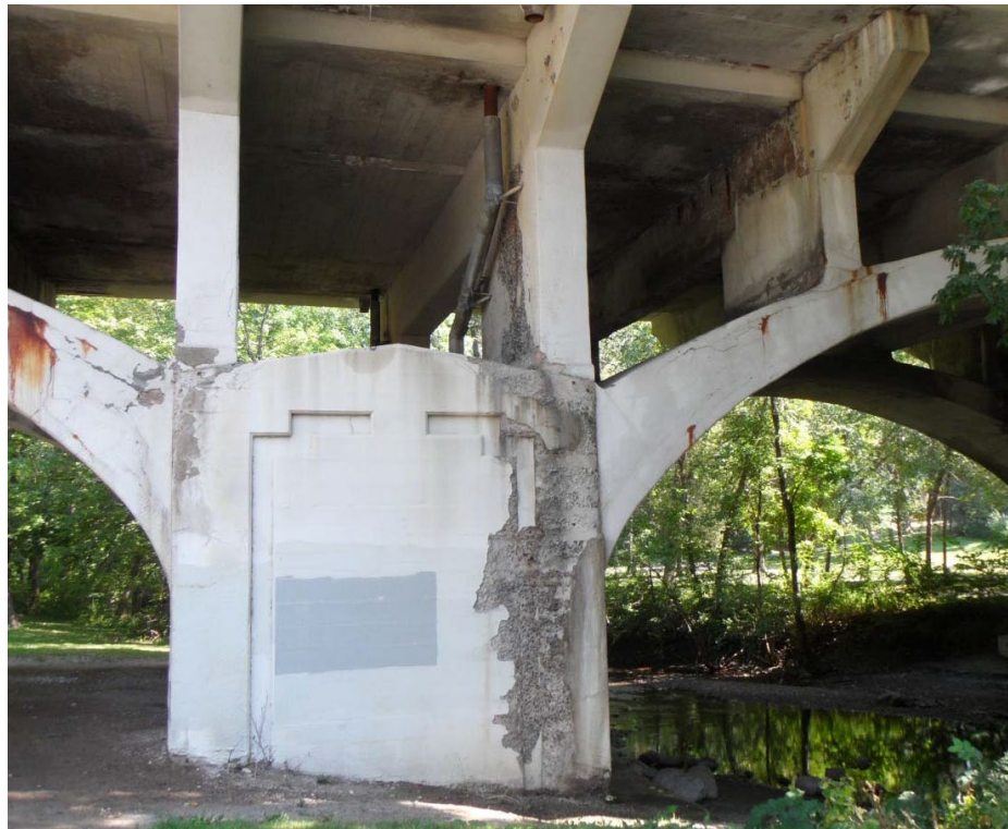
Figure 11: West Pier at Creek (2012)
