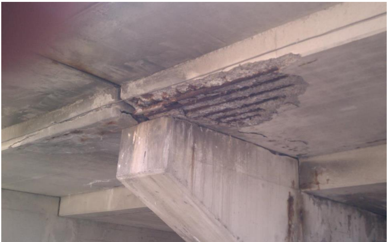
Figure 5: Deck Delamination (2011)
