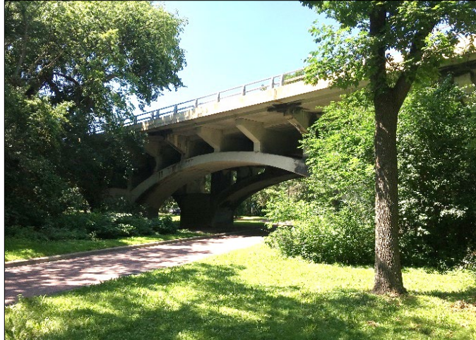
Minnehaha Parkway under Nicollet Ave. Bridge
