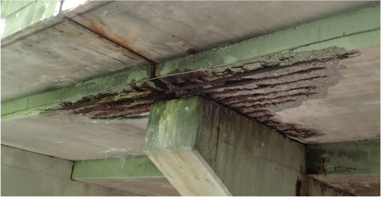
Figure 6: Deck Delamination (2019)
