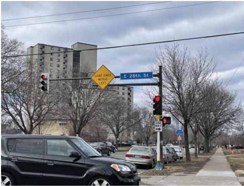
(Above) Several signals along the corridor are past their useful life and are in need of replacement, such as the signal at Portland and 28 th St which was first constructed in 1956.
