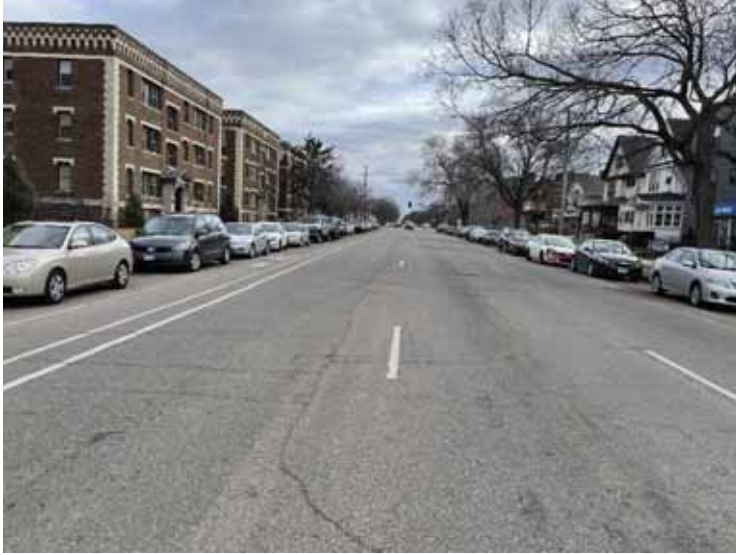
View of existing 3-lane, one way configuration and existing on-street bicycle facility on Portland Ave at 28 th St facing south.
