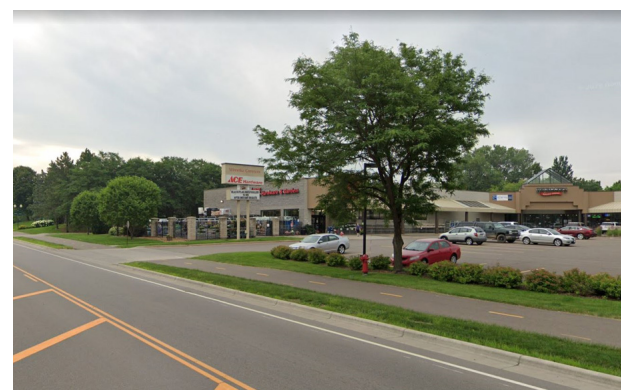
Typical regional trail along road through a more developed setting: The above photo shows an example of what the trail will look like following construction.
