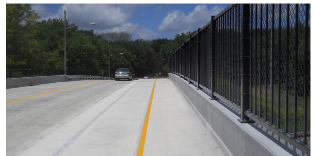
▲ Typical regional trail across existing highway overpass: The above photo shows how bridge redecking would create space to accommodate the regional trail on the east side.
