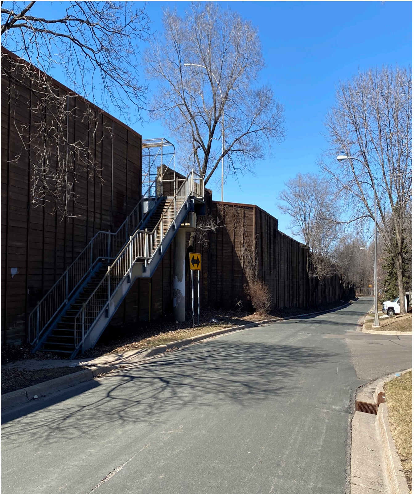
Existing site condition photo
