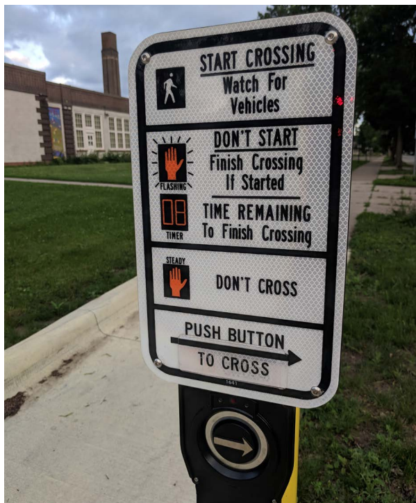
Figure 4-8: Accessible Pedestrian Signal (APS) push button
