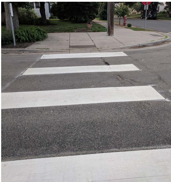
Figure 3-18: Minneapolis' standard pattern for crosswalk markings is the Minneapolis Zebra
