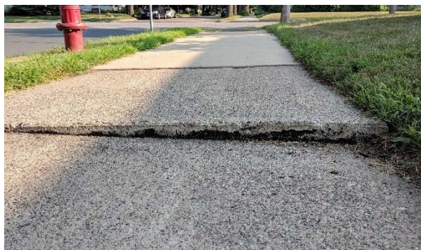
Figure 2-7: Raised panels on sidewalks and broken sidewalks present a barrier to safe walking and rolling
