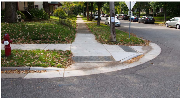
Figure 3-2: Combined Directional Pedestrian Curb Ramps provide two separate ramps at each corner
