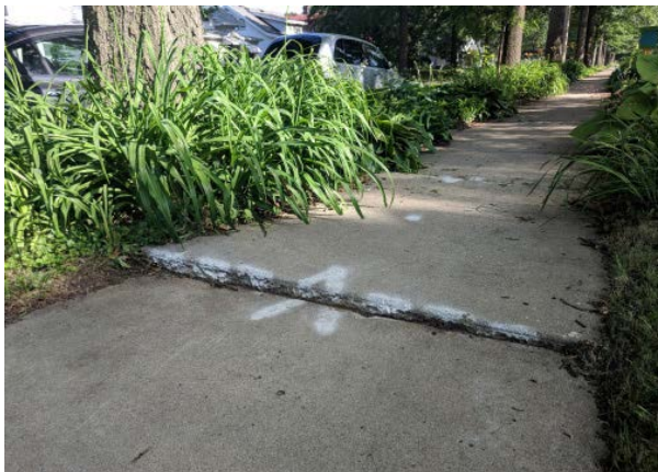
Figure 4-11: Uneven sidewalk
