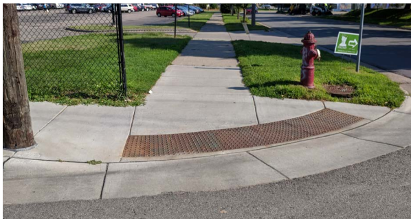
Figure 3-3: Fan Ramps or Depressed Corner Ramps provide one ramp to cross the street in either direction
