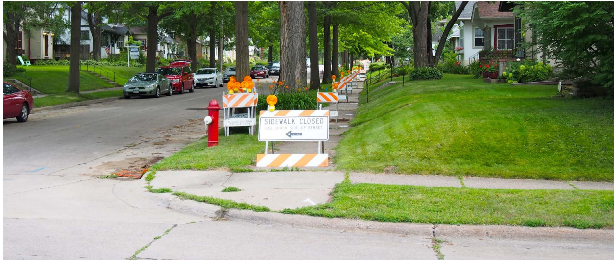
Figure 3-23: Sidewalk with “Sidewalk Closed” signage while sidewalk is being repaired
